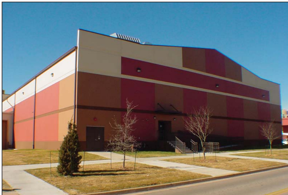
The new Integration Support Facility at Tinker Air Force Base. Work done in the facility is classified, so it displays secure construction features such as a lack of windows.
