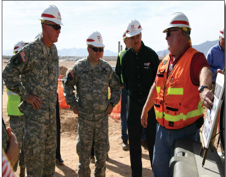
Lt. Gen. Robert L. Van Antwerp, Col. Christopher Martin, and Troy Collins are briefed by David Buchanan, Biggs Area Office, about the progress of ongoing construction at Biggs Army Airfield.
