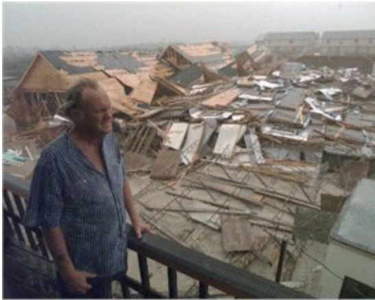
Jim Larkin looks toward the ocean as he stands on the deck of his condo Saturday. Below him is a four-story condo that collapsed that had been under construction (AP Photo/July 21, 1997)
