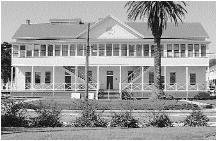
Building 36 after rehabilitation. Photo by Robert Wallace.
