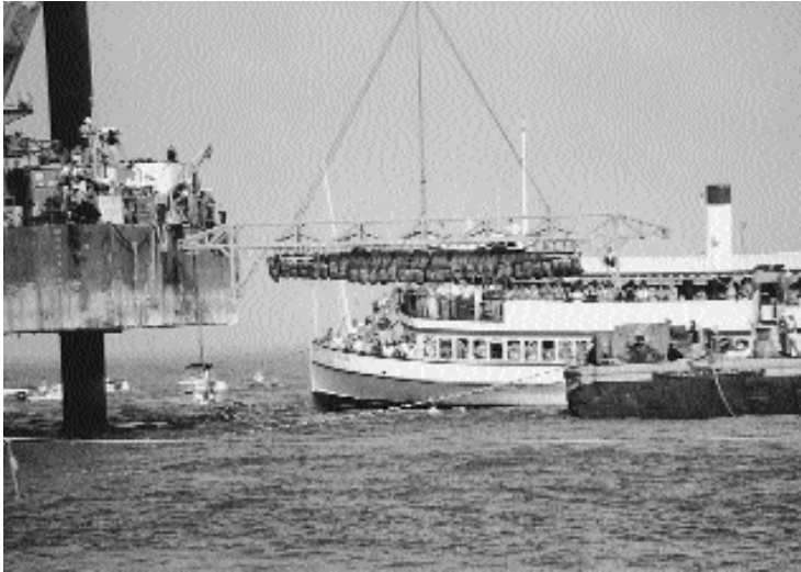
August 8, 2000 8:45 a.m., Hunley and frame are safely lifted from the bottom and placed on the transport barge. Photo courtesy Tim Smith, NPS.
