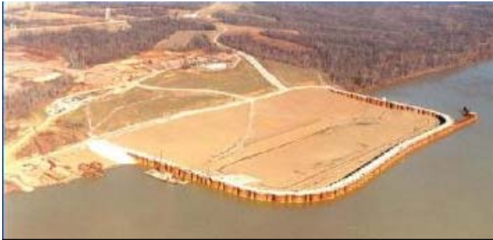
Figure 5. Cofferdam at Olmstead Dam.
