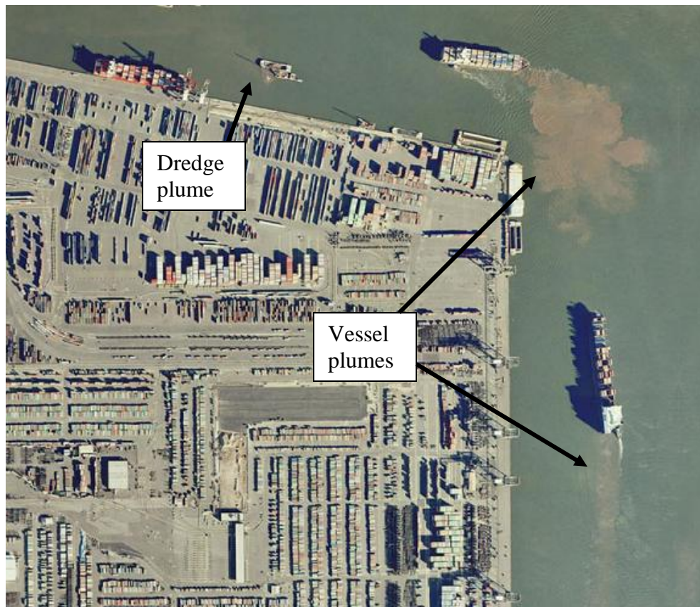
Figure 1. Comparison of dredge and vessel induced turbidity in Elizabeth Channel 28 Dec 2001.
