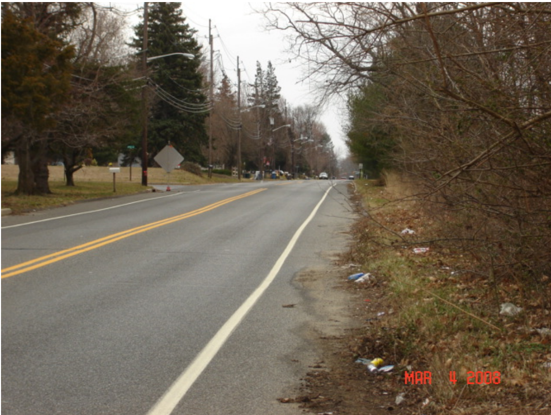
Lower Landing Road, facing south
