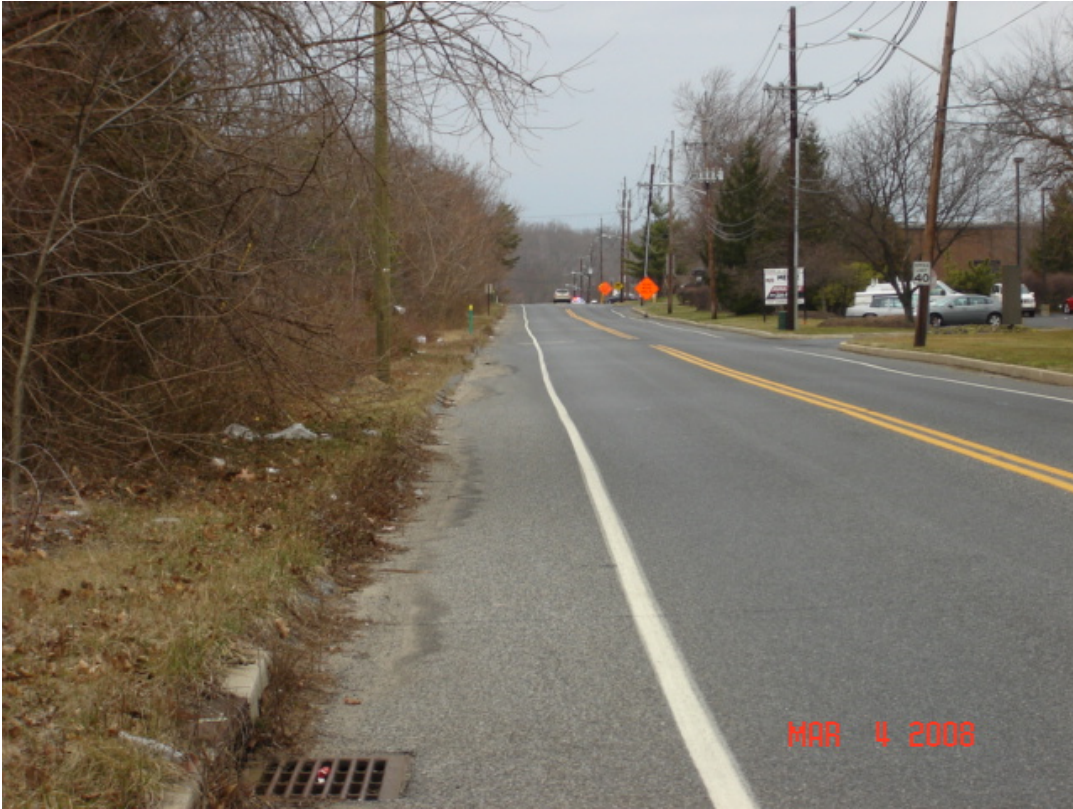
Lower Landing Road, facing north
