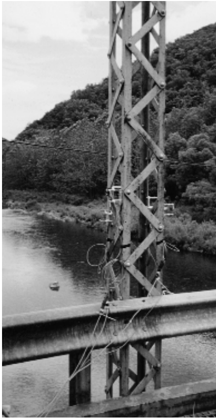
Detail of vertical member (labeled U11-L11 in drawing on next page), with strain gauges installed for load testing. Photo by author, 1998.
