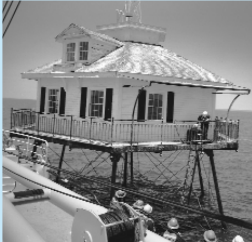
White Pine conducting maintenance work on midbay lighthouse in Mobile Bay. Crew is removing ladder from lighthouse for repairs. White Pine crane and winch are in foreground. To avoid getting in the way of a very active crew, this shot had to be taken without a tripod. Bright light enabled stopping down for depth of field while maintaining a relatively fast shutter speed.
