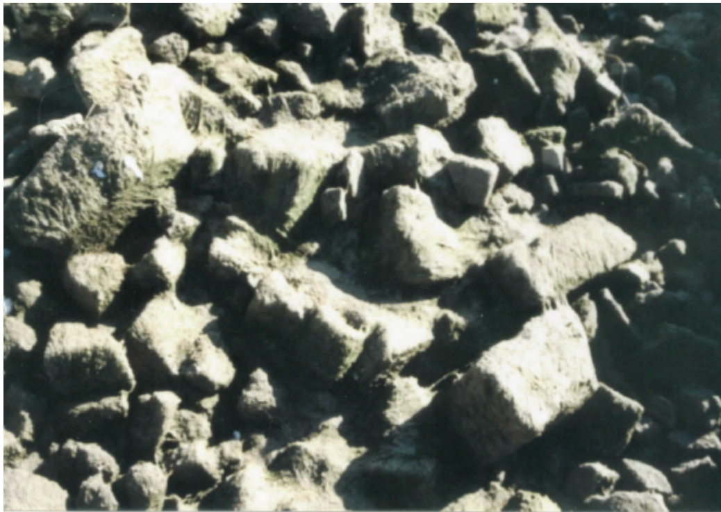
Figure 6. Algae covered riprap. This quartzite riprap had been submerged for about 3 months. Rock size ranges from more than 1 foot to about 3 inches. Algae covered rock is unsuitable substrate for spawning sturgeon.
