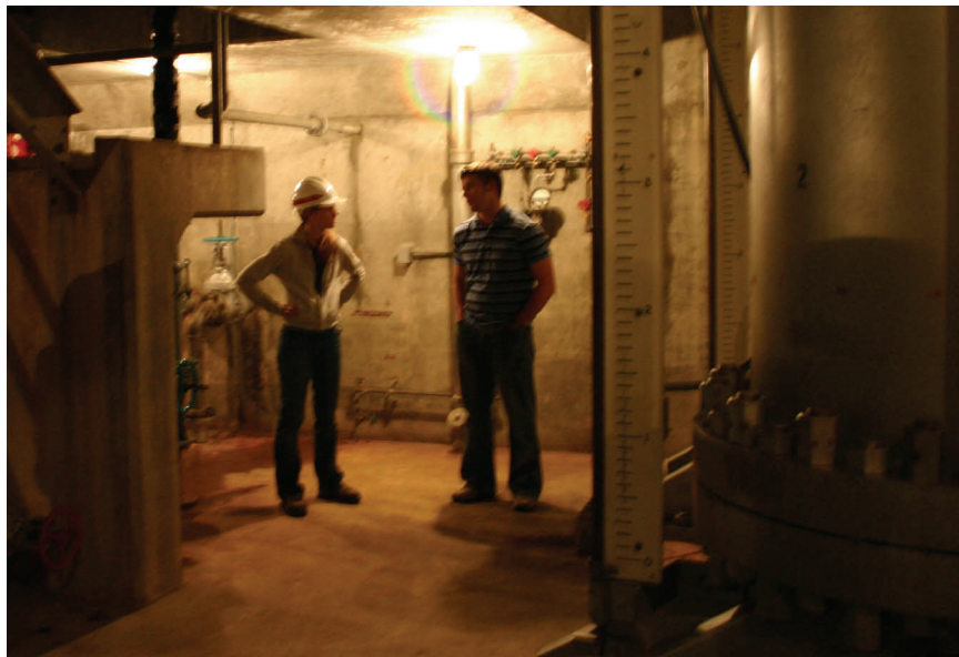
EITs DISCUSS CONDITIONS IN THE INTAKE TOWER AT COUGAR DAM, OREGON
