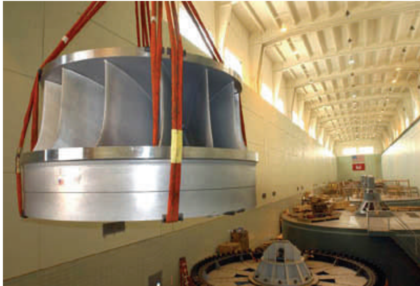
A NEW FRANCIS TURBINE RUNNER INSTALLATION AT J. STROM THURMOND DAM, SOUTH CAROLINA
