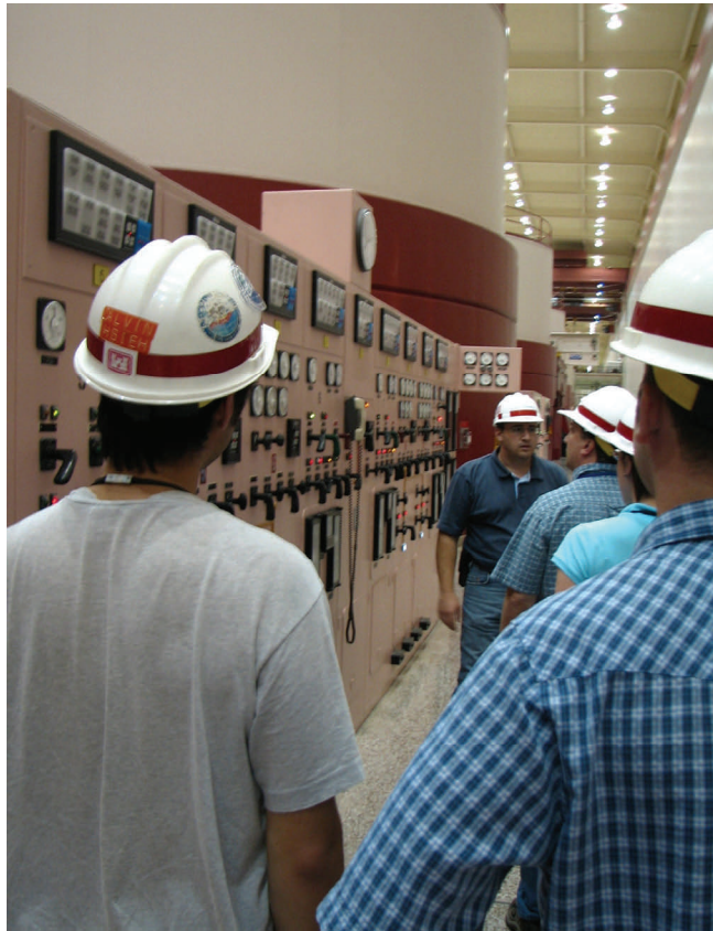
EITs OBSERVE A GOVERNOR CONTROL PANEL AT CHIEF JOESPH DAM, WASHINGTON
