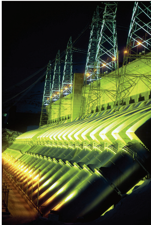
PENSTOCKS LIT DURING THE NIGHT AT CHIEF JOESPH DAM, WASHINGTON
