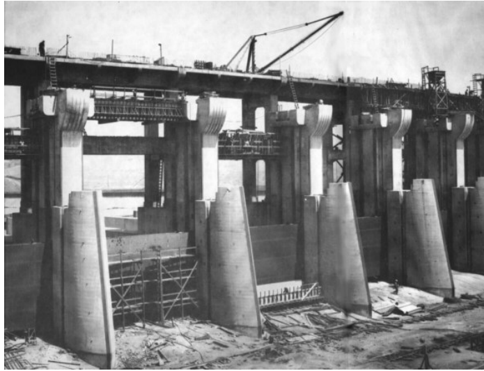
CONSTRUCTION OF FORT PECK DAM, MONTANA
