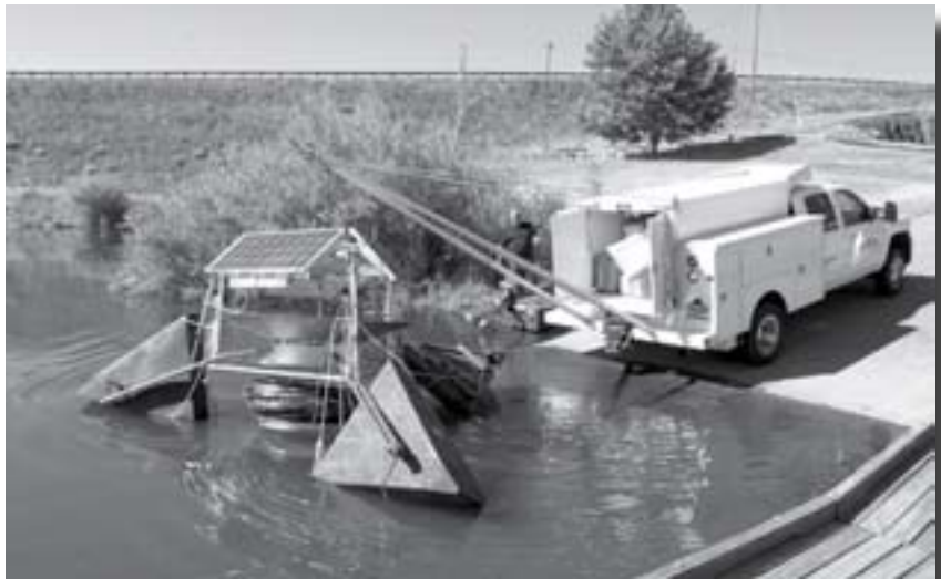
One of the two long distance circulators is backed down the ramp into Willow Creek Reservoir as part of a pilot study to manage harmful algae blooms.
