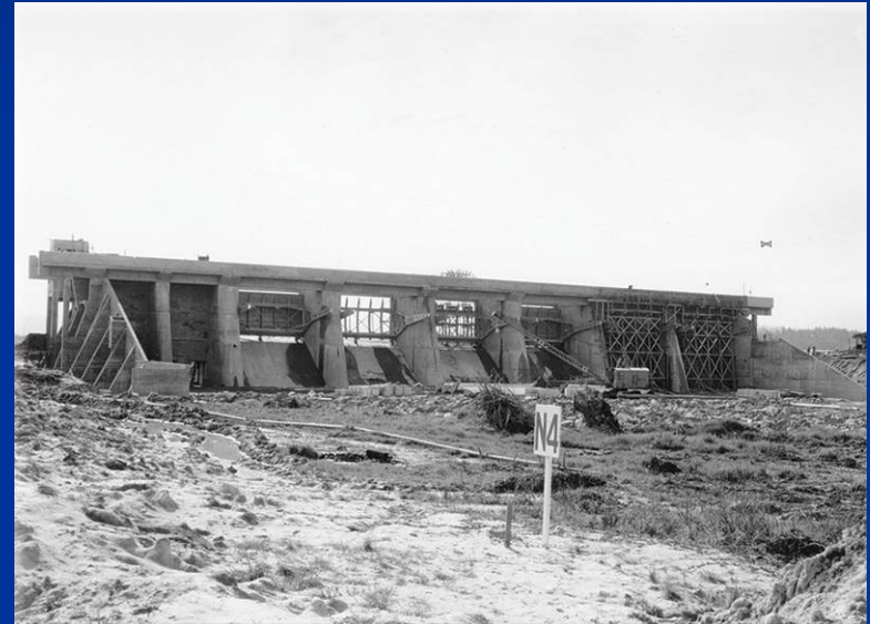
Fern Ridge Dam construction
