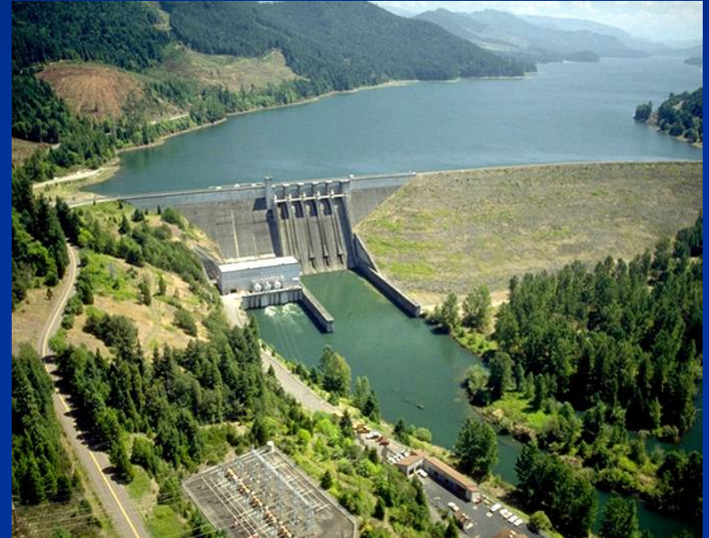
Lookout Point Dam
