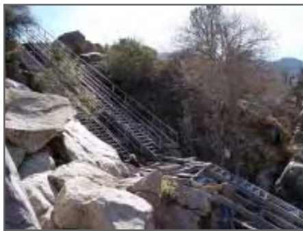
A boat slide project, under construction at the Lower Kern River.
