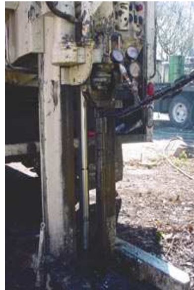
Figure 6. EZVI remediation technology in process.
