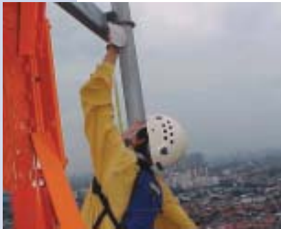
An IBB antenna maintenance technician, known as a "rigger," works on an IBB antenna tower in Indonesia.
