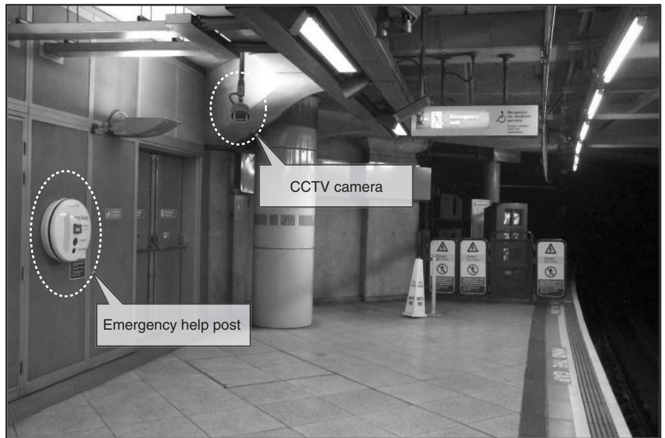
Figure 9: Security Design Elements Incorporated into London's Underground
