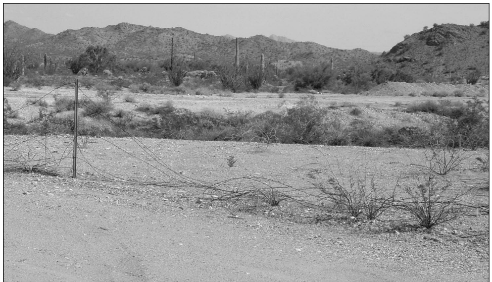
Figure 7: International Border Fence on Federal Land in Arizona, Presumed Damaged by Illegal Aliens or Smugglers
