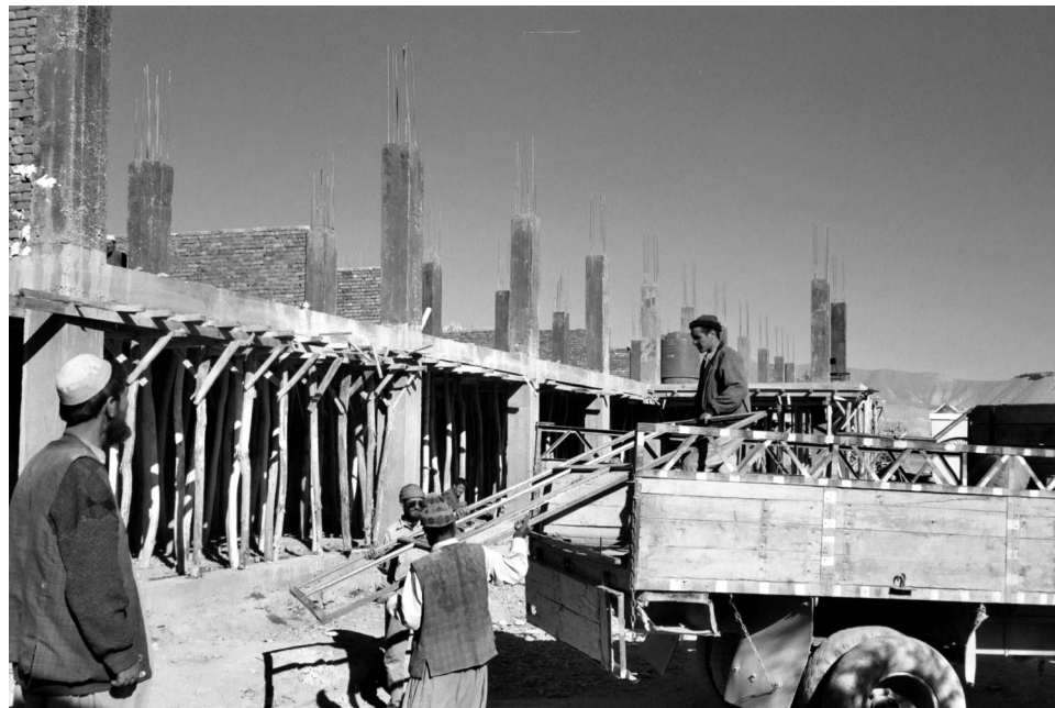
Figure 9: PRT-Funded Construction of Provincial-level College in Bamian Province, Afghanistan
