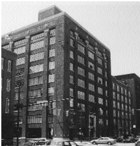
The Otis Terminal Warehouse, listed as part of the Cleveland Warehouse District, is a recently completed federal rehabilitation tax incentive project. Photo courtesy Sandwick Architects.
