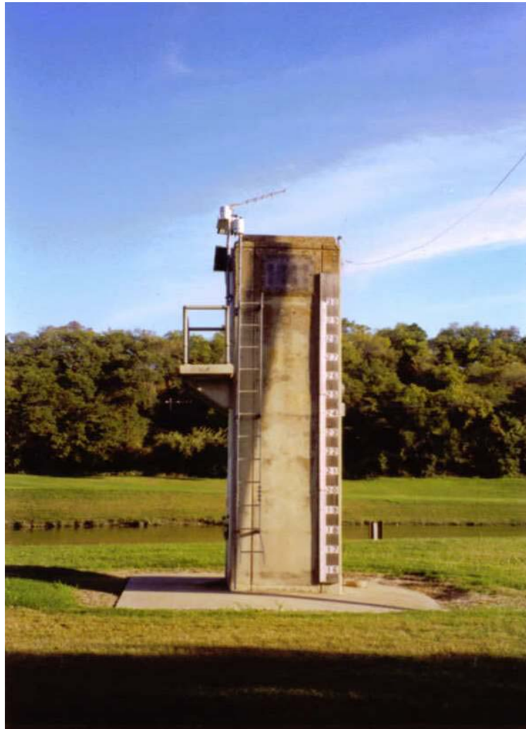
Figure 47. USGS river gauge located near Nutt Dam (Property Number 104).
