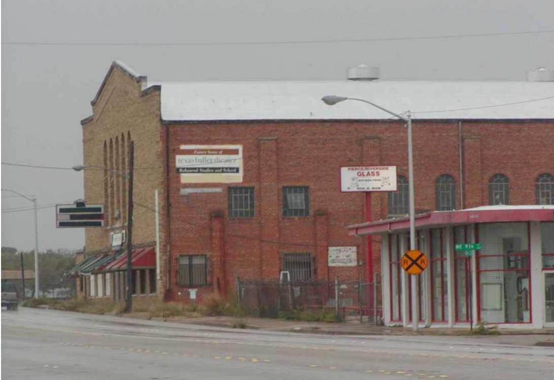
Figure 29. Former KKK Hall and Ellis Pecan building (Property Number 62).
