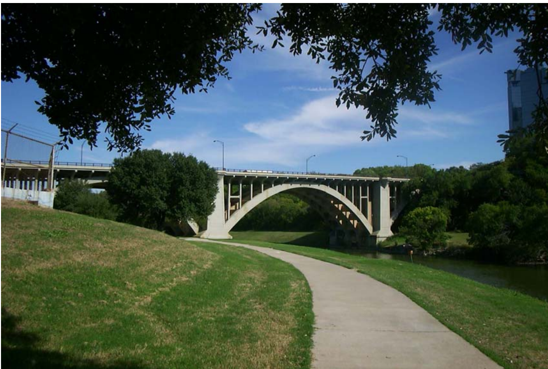
Figure 50. Paddock Viaduct (Property Number 103).
