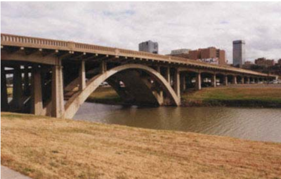
Figure 51. Henderson Street bridge (Property Number 101).
