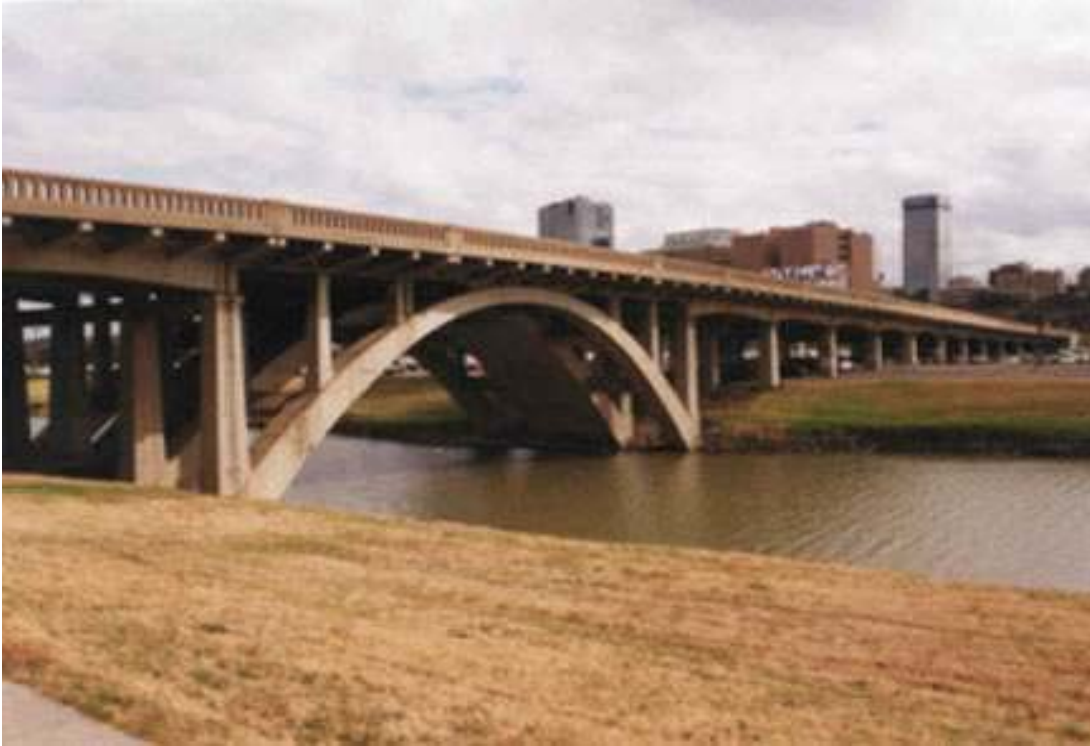
Figure 68. Henderson Street Bridge (Property Number 101).
