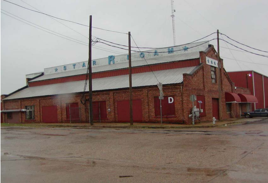
Figure 81. Machine Shop, 1107 North Calhoun (Property Number 65).
