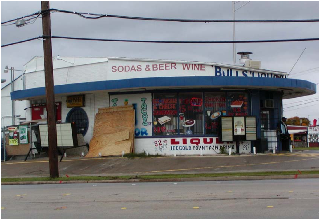
Figure 17. Package store on North Henderson (Property Number 87).
