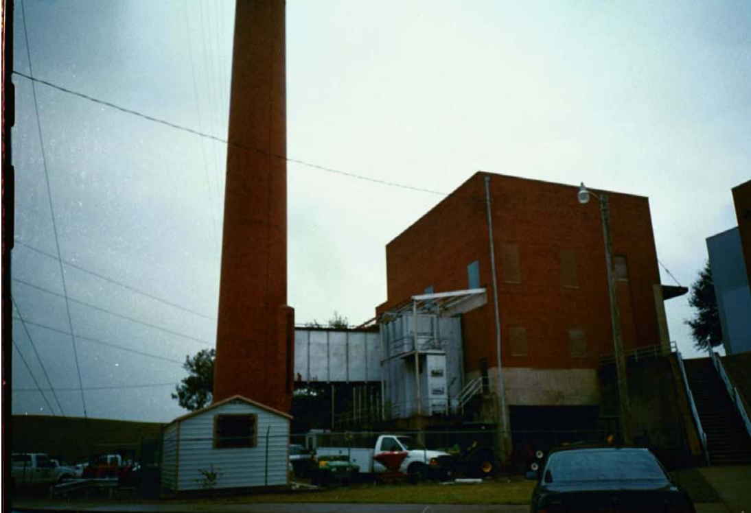
Figure 84. Stack and boiler house of the Fort Worth Water Department, 900 Woodward (Property Number 96-A).
