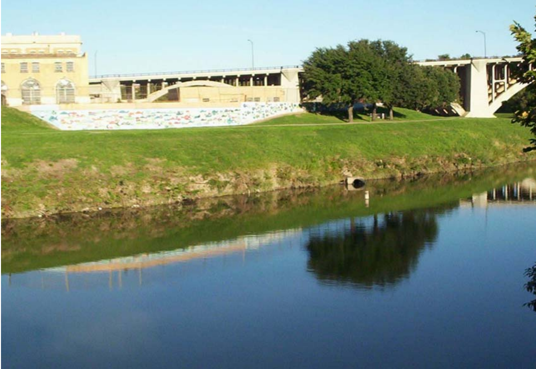
Figure 65. Floodwall with fill added along the base (Property Number 104).
