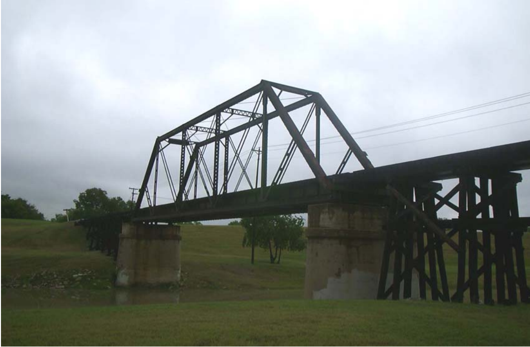
Figure 69. St. Louis, San Francisco and Texas Railway Bridge (Property Number 102).
