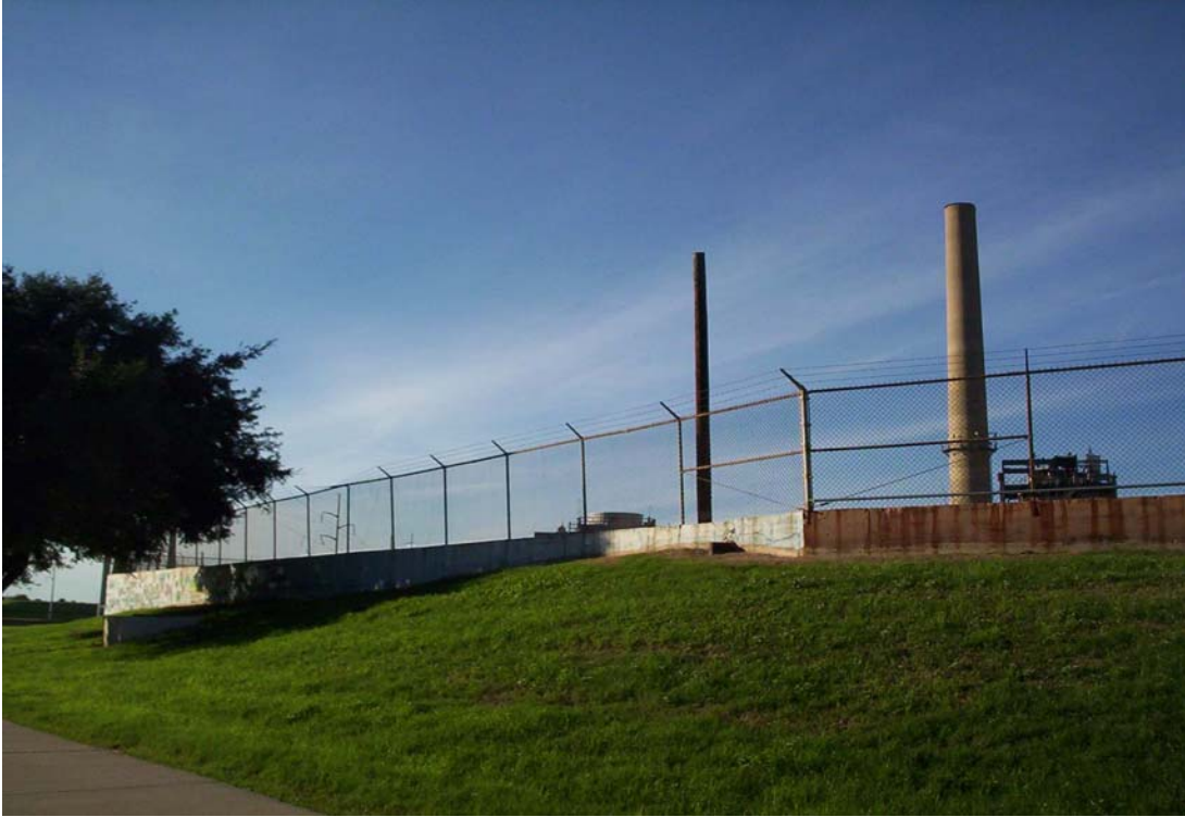
Figure 37. Flood wall of the city's electric power plant.
