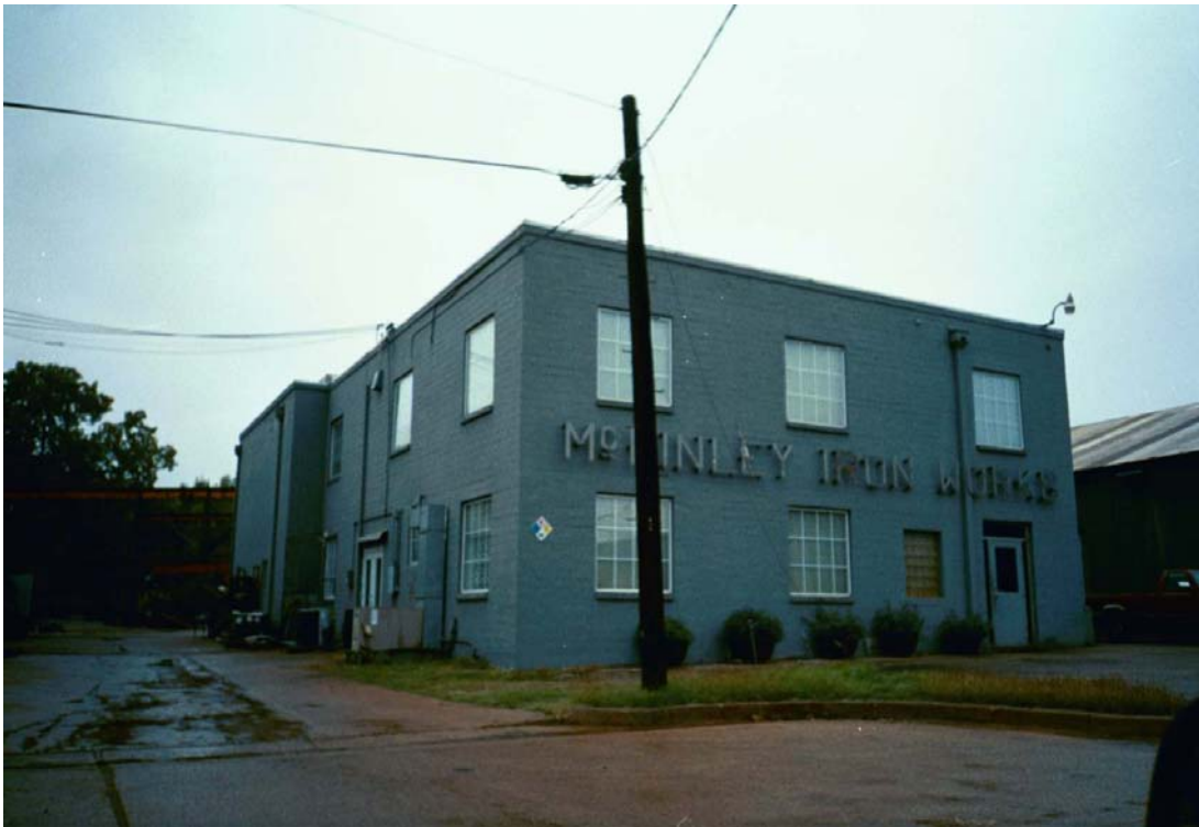
Figure 27. McKinley Iron Works (Property Number 47).
