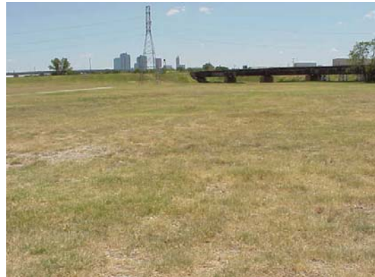
Site 161, south view.
