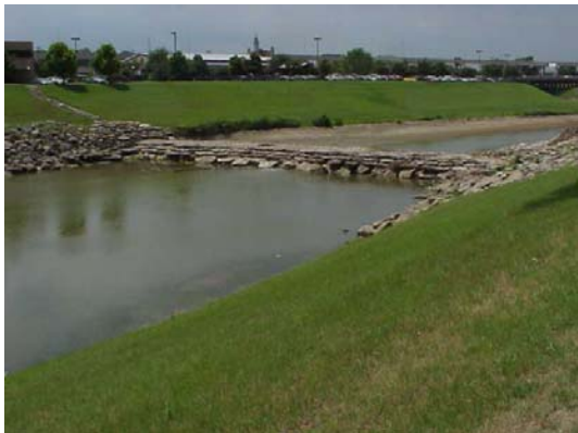
Low water dam at Trinity Park.
