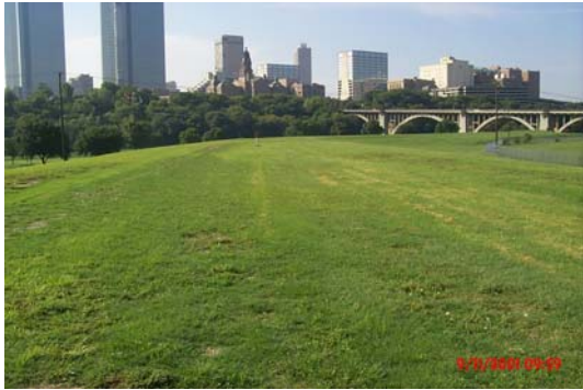
Levee along the north side of the river east of the Main Street Bridge.
