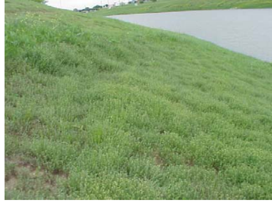
Site #112, south view.
