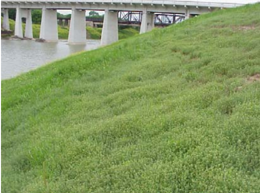
Site #112, north view.
