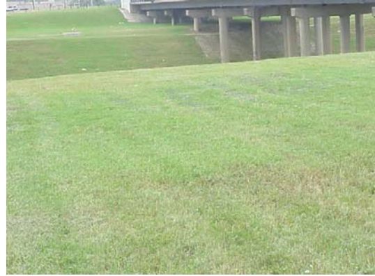
Site 131, south view.
