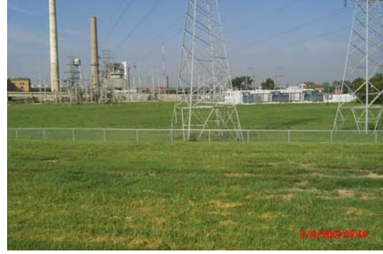
Old Power Plant north of the Main Street Bridge.
