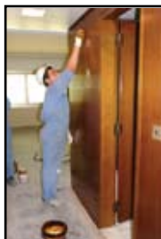
An Iraqi worker stains teak paneling in a guest room of the Al Rasheed Hotel. A $5.16 million renovation of the hotel is nearing completion in Baghdad.
