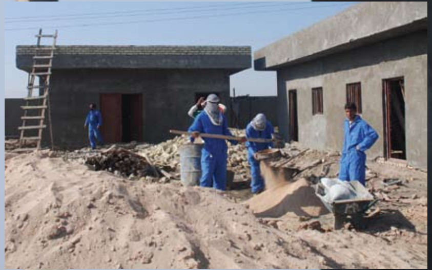
Workers mix plaster for the al-Takadoom plant.
