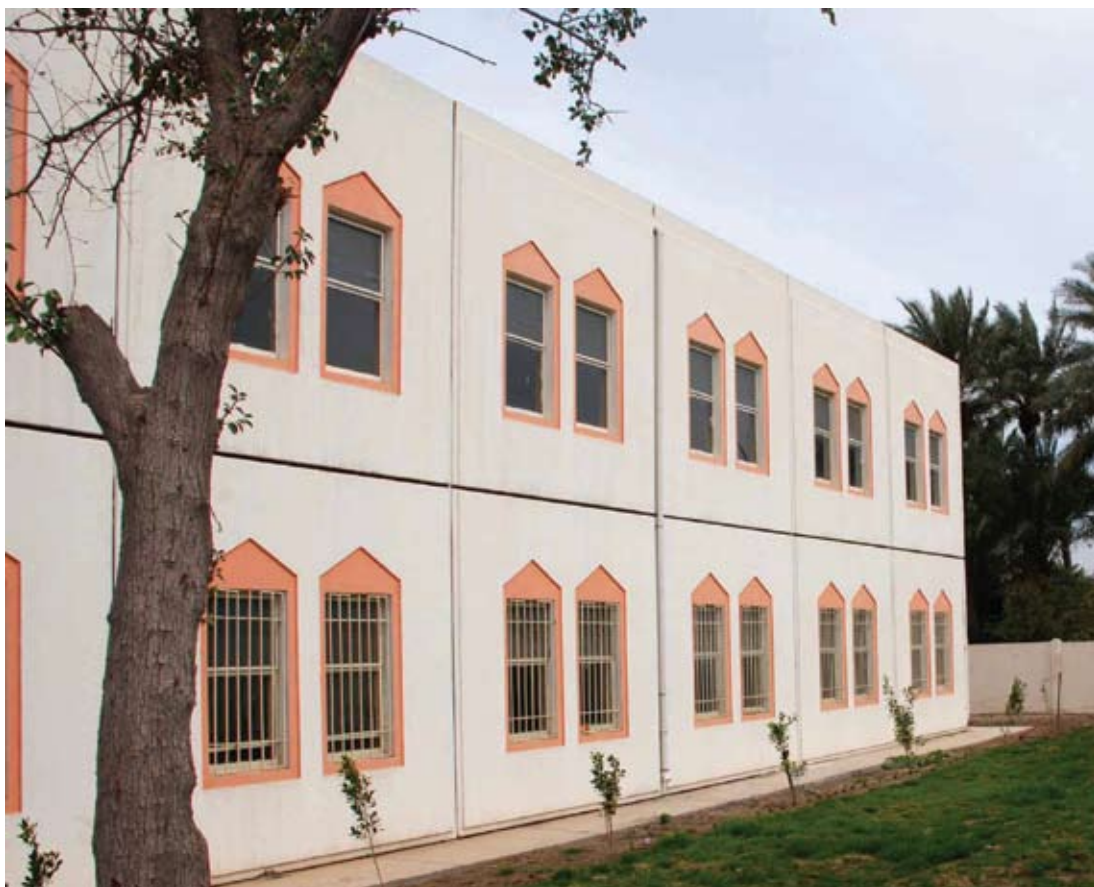
Exterior work on al-Qudis school included painting and grounds work.
