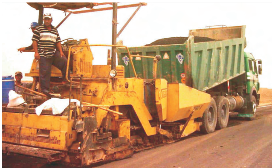
A new all-weather asphalt road now leads to the landfill.
