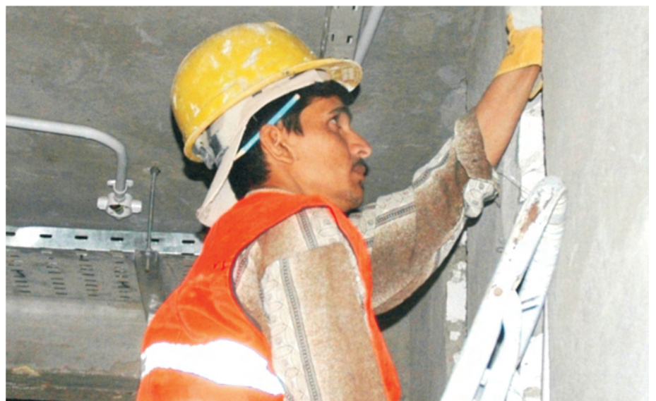
Iraqi electrician installing wiring in the $1.4 million courthouse.
