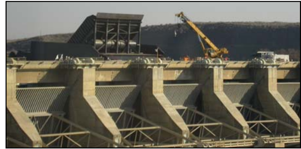
A spillway weir was installed at Ice Harbor Dam in February 2005.
