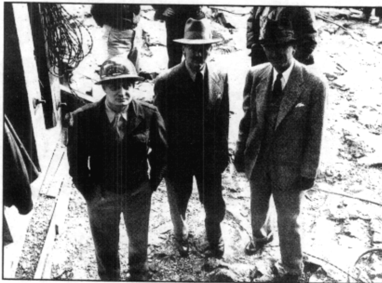
Col. William Whipple, center, first Walla Walla District Engineer, at McNary Dam construction site, 1948.
