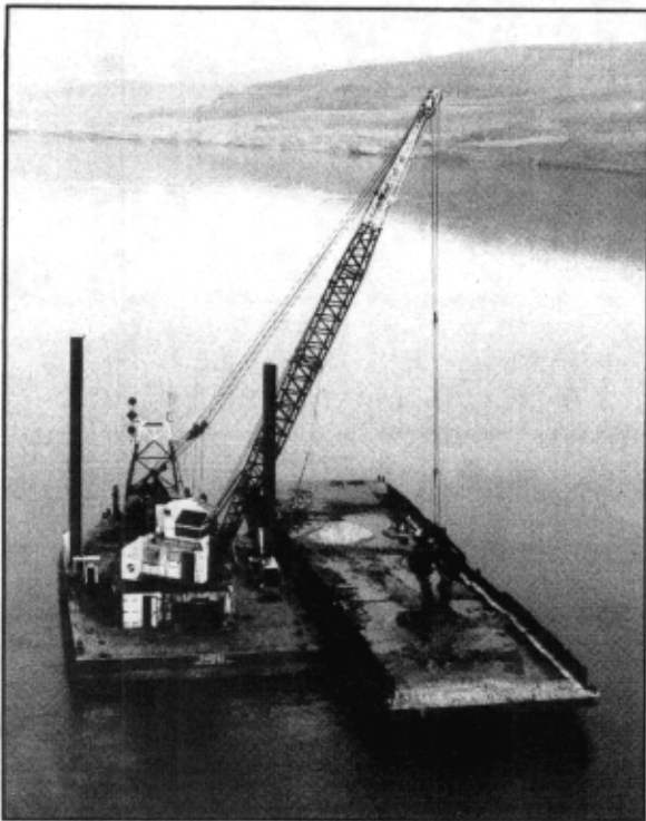
Dredging behind Lower Granite Dam, where most sediment accumulates.
