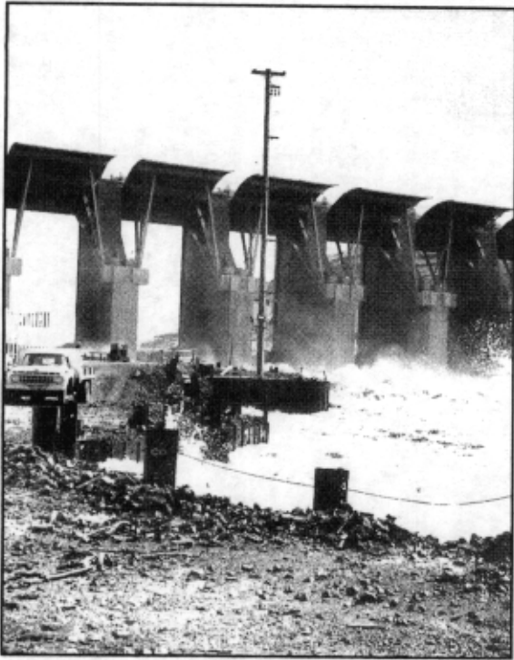
Construction at Lower Monumental Dam, 1960s.
