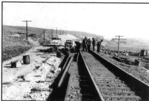
Relocation track for Spokane, Portland & Seattle Railroad.
