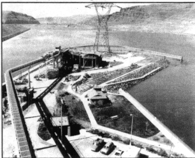
Juvenile fish bypass facilities at Little Goose, 1990; at left: looking east at entire length of bypass system; at lower left: bypass channel as it descends to the outfall chute; at lower right: west end of bypass channel with outfall chute to right.
