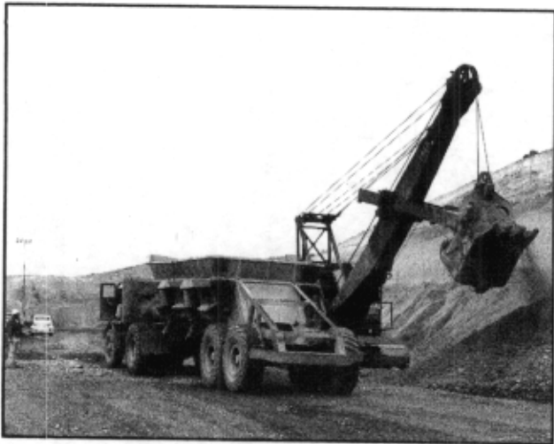
Excavation at Ice Harbor dam site, July 1956.
