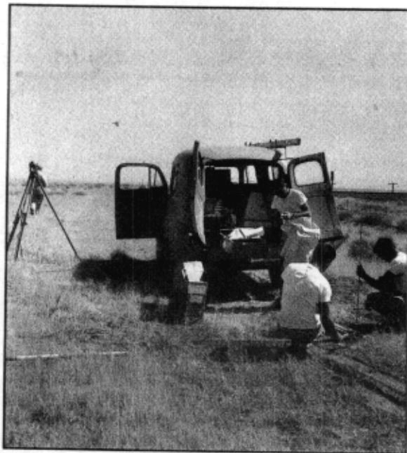
Surveying for access road to Ice Harbor construction site. August 1955.
