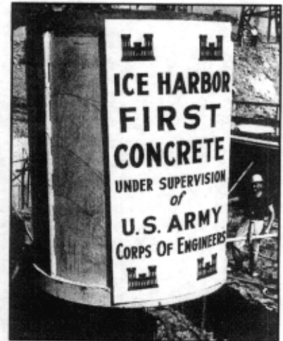
Construction of Ice Harbor finally got underway in 1956.
