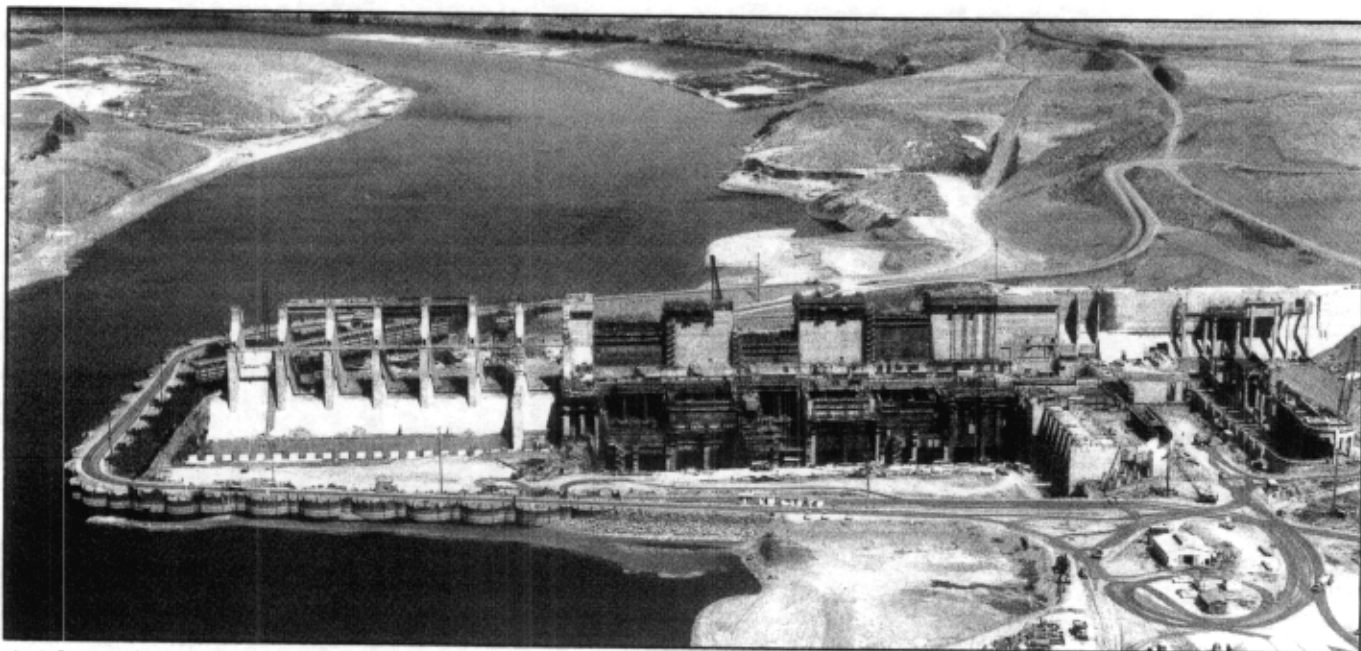
Aerial view of south shore construction.
