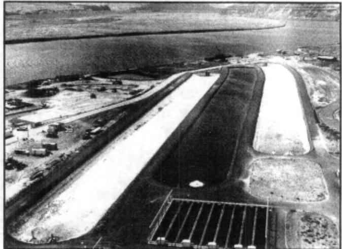
Lyons Ferry Fish Hatchery construction, 1983.
