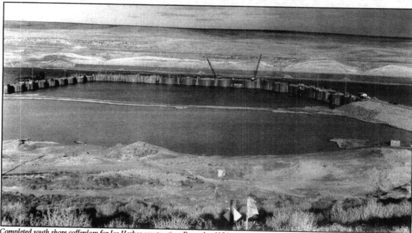
Completed south shore cofferdam for Ice Harbor construction, December 1956.
