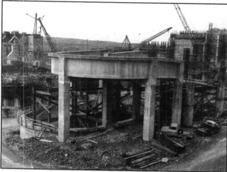
Fish ladder construction, May 1958.
