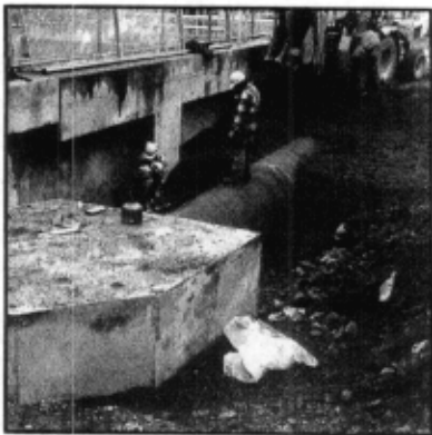
Backfilling around original fingerling bypass pipe, Little Goose Dam, 1979.
