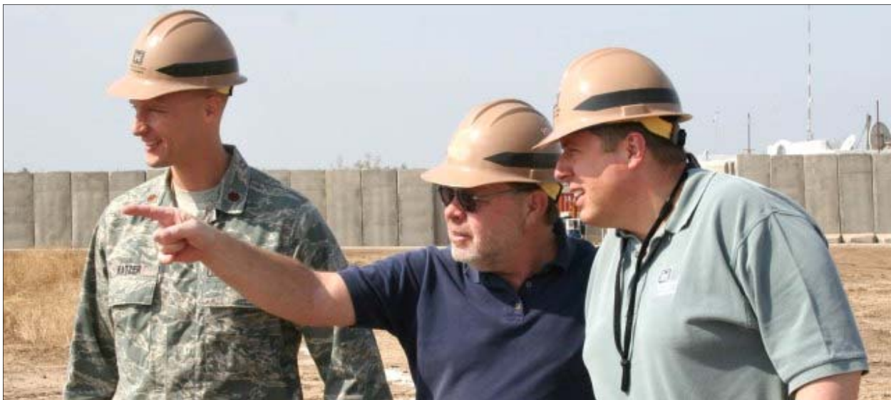
Maj. Dee J. Katzer (left), Construction Representative Tommy Nason, and Project Manager Steve Farkus view the site where a new $30 million 60,000 sq. ft. dining facility is being constructed at Camp Delta in Wassit Province. (USACE photo)
