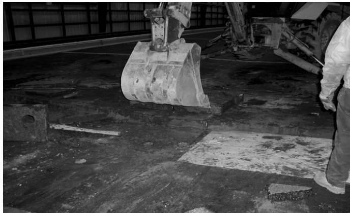
FIGURE 9. P-401 REMOVAL
