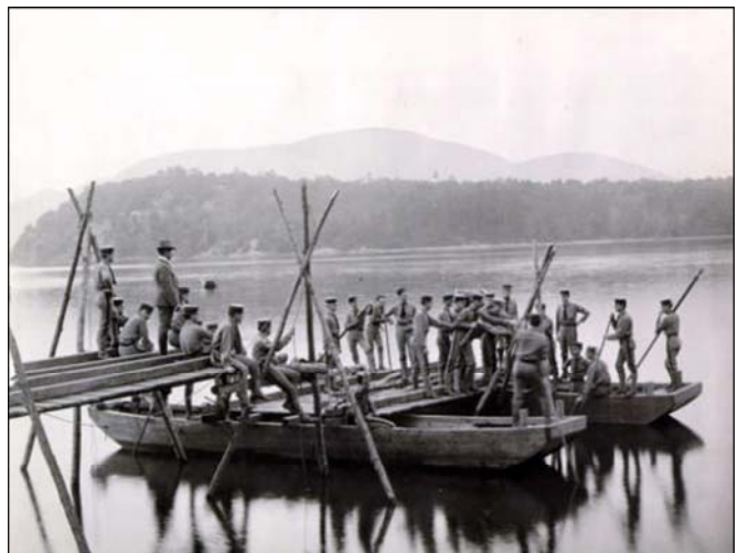
Engineering has long been a strength of the USMA curriculum. Here cadets build a trestle bridge during a military engineering class, ca. 1906 (USMA Archives).
