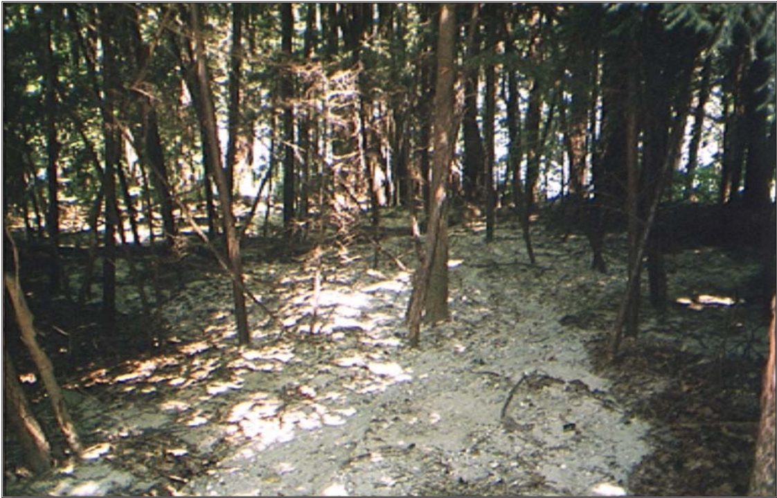
Sand and gravel washed from a dirt road after a severe rainstorm is captured by a forested buffer. The nearby lake is in the background. Source: BRPC archive, 2000.
