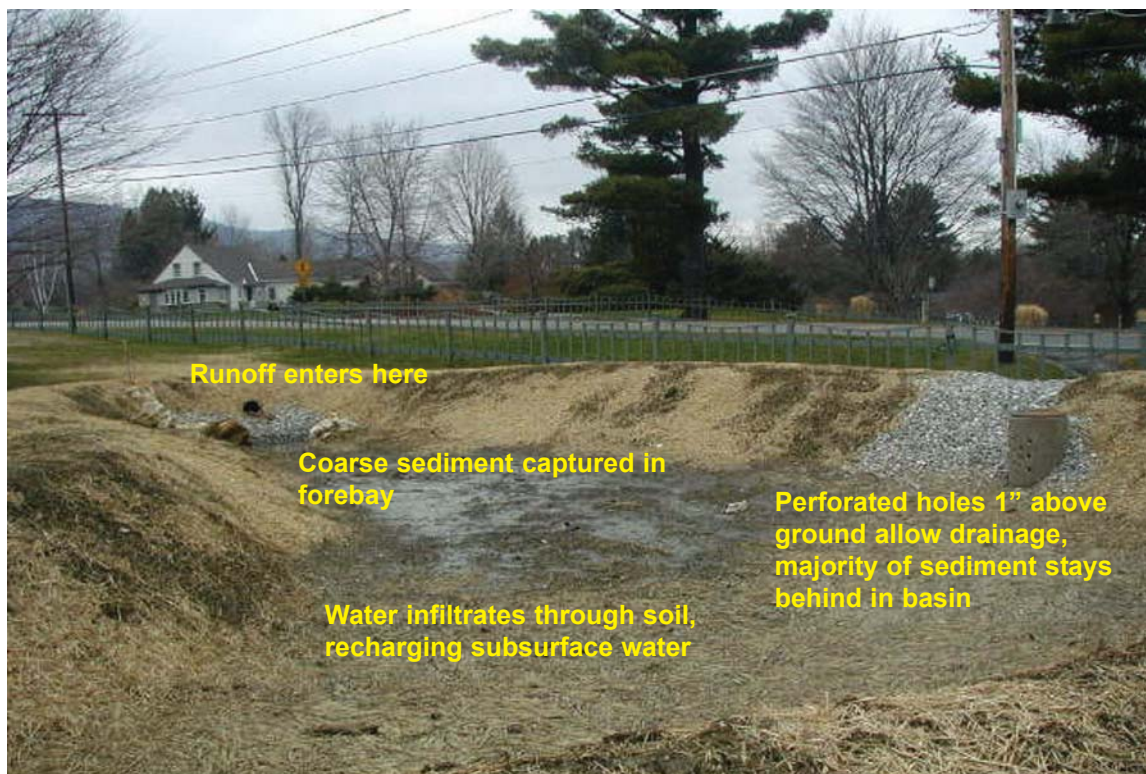
Construction of a retention basin, which is being converted into a wetland garden. It captures sediment and other pollutants.
