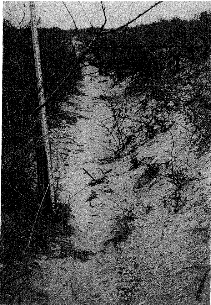
Fig. 3. Gully between Walnut Gulch 101 and 103 runoff-measuring stations.
