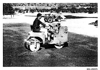
Figure 10.—Compacting a catchment apron with a self-propelled vibrating drum roller.
