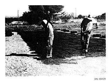
Figure 16.—Gravel placement on gravel-covered membrane catchment treatment.
