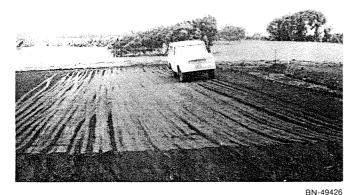
Figure 11.—Compacting a catchment apron with a rubber-tired vehicle.
