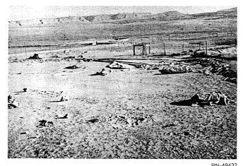
Figure 19.—Butyl rubber catchment destroyed by wind.
