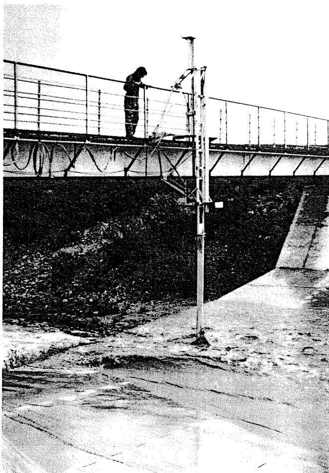
FIGURE 21.—Instrument carriage and velocity meter probe in use at flume 63.006, August 10, 1976. BN-48656
