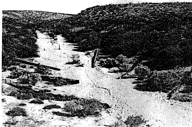
FIGURE 31.—Prototype control dikes at flume 63.003 after large storm flow in early dike evaluation at Walnut Gulch Watershed. BN-48660
