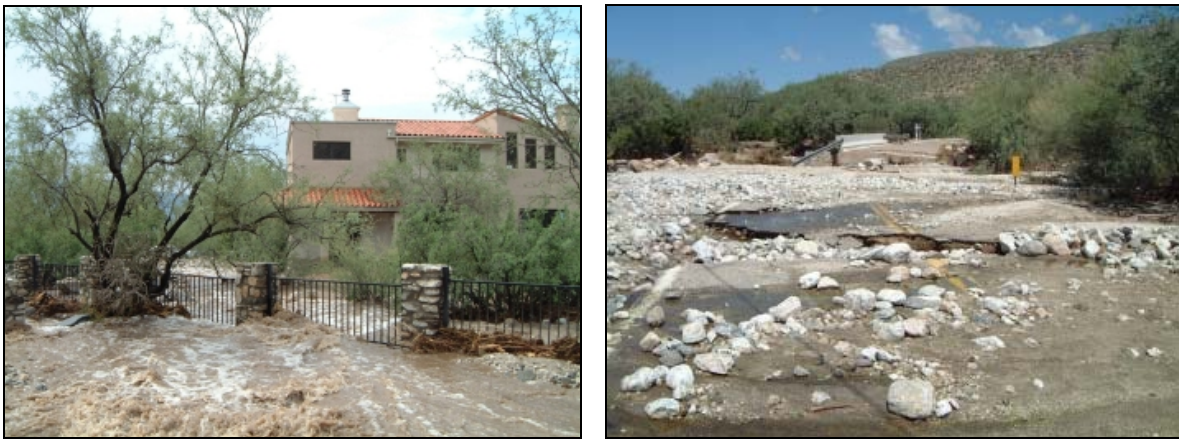
Figure 20. Photographs from an unusually large flood event in an ephemeral stream that damaged roads and bridges, and flooded nearby homes, Tucson, Arizona, July 31, 2006.
