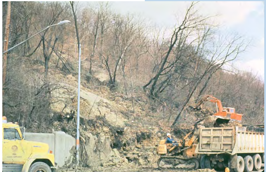
Figure 12. Earthflow material being removed by a highway crew along the Columbia Parkway, Cincinnati, Ohio. Hamilton County, in the metropolitan Cincinnati area, experienced an average annual economic loss of $5.80 per person (1975 dollars) between 1973 and 1978, the highest calculated per capita loss of any municipality in the United States. Photograph courtesy of the U.S. Geological Survey.
