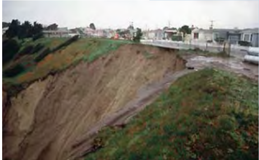
Figure 13. Gully retreat threatening evacuated houses in Daly City, a suburb of San Francisco, California, following the storm of February 2–3, 1998. Landslide and mudslide activity was extensively reported in the news media following heavy rains on February 2–3, 1998. A number of scattered, slow-moving landslides had been active over the weeks prior to the storm in San Francisco, Oakland, and elsewhere in the San Francisco Bay region. As most of the area experienced about 200 percent of normal rainfall in the winter of 1998, these landslides were probably related more to the wet winter and less to the effects of this particular storm. However, based on limited ground reconnaissance, scattered slope movements directly related to the storm did occur. Debris flows directly triggered by the storm affected a number of homes and properties. From U.S. Geological Survey web site http://landslides.usgs.gov/html_files/landslides/reconrpt.html , 1998, accessed July 29, 2002. Photograph by Steve Ellen, U.S. Geological Survey.
