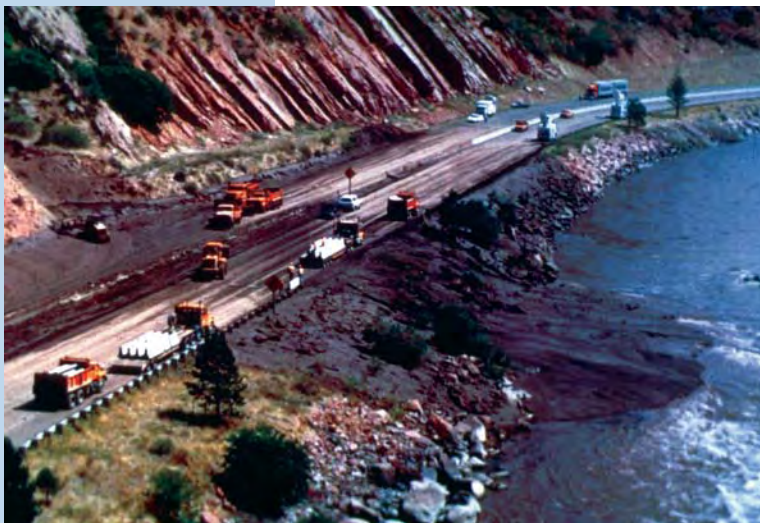
Figure 2. Debris flows like this one near Glenwood Springs, Colorado, in 1994 are a consequence of heavy rainfall on previously burned hillsides. In addition to personal injuries and damage to 30 vehicles engulfed by these flows, transportation along the Interstate 70 corridor was brought to a standstill for a day, and business and emergency operations in the Glenwood Springs area were seriously impeded. Photograph by Jim Scheidt, U.S. Bureau of Land Management.
