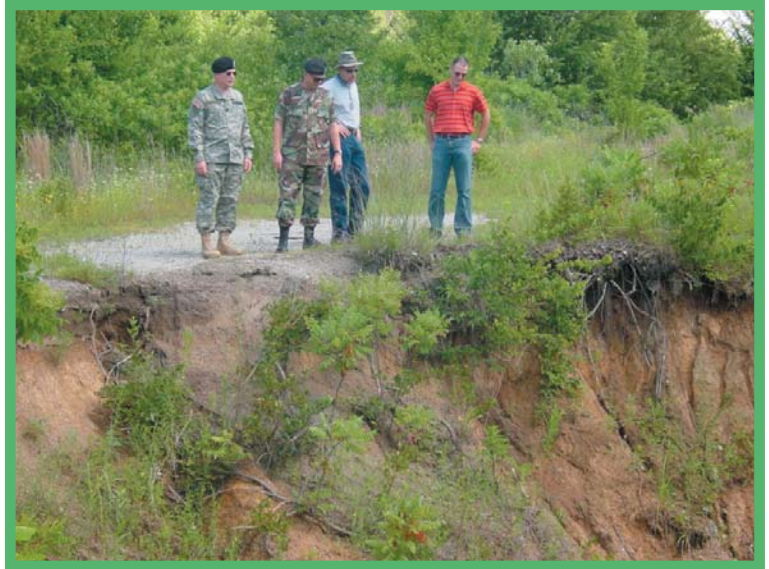
Gen. Jeffrey Dorko, Southwestern Division commander; Col. Miroslav Kurka, Tulsa District commander; Jim Martel; and Adam Crisp, Tar Creek Project Delivery Team members, inspect a sinkhole in the Picher/Cardin area.
