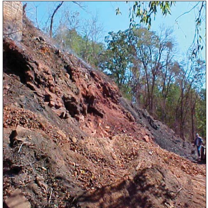
The contractor is dwarfed by the gob pile created by miners in the late nineteenth/early twentieth century on land now managed by the Corps at Eufaula Lake.
