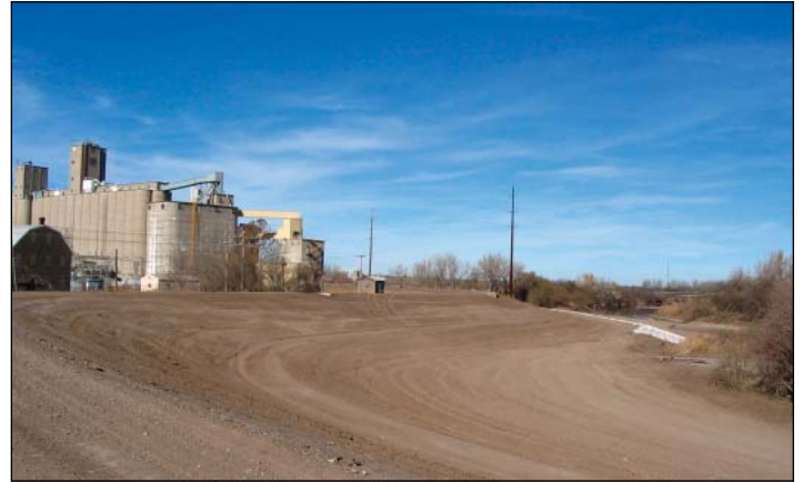
A view of the levee at the Archer Daniels Midland plant.
