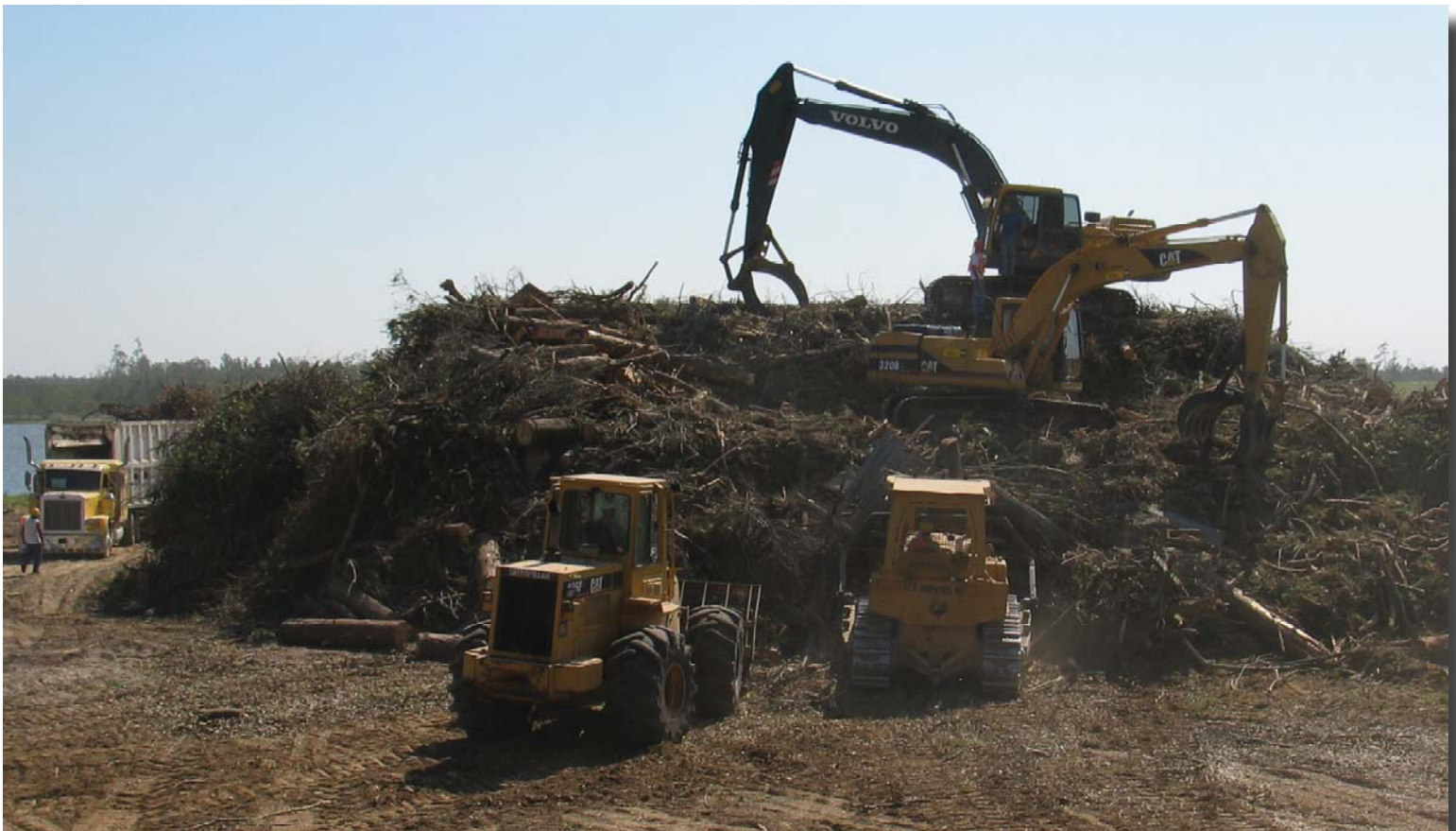
A debris reduction site in Southeast Texas.
