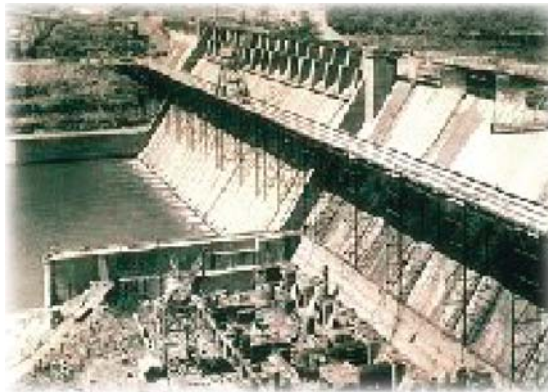
Photo courtesy of Little Rock District
