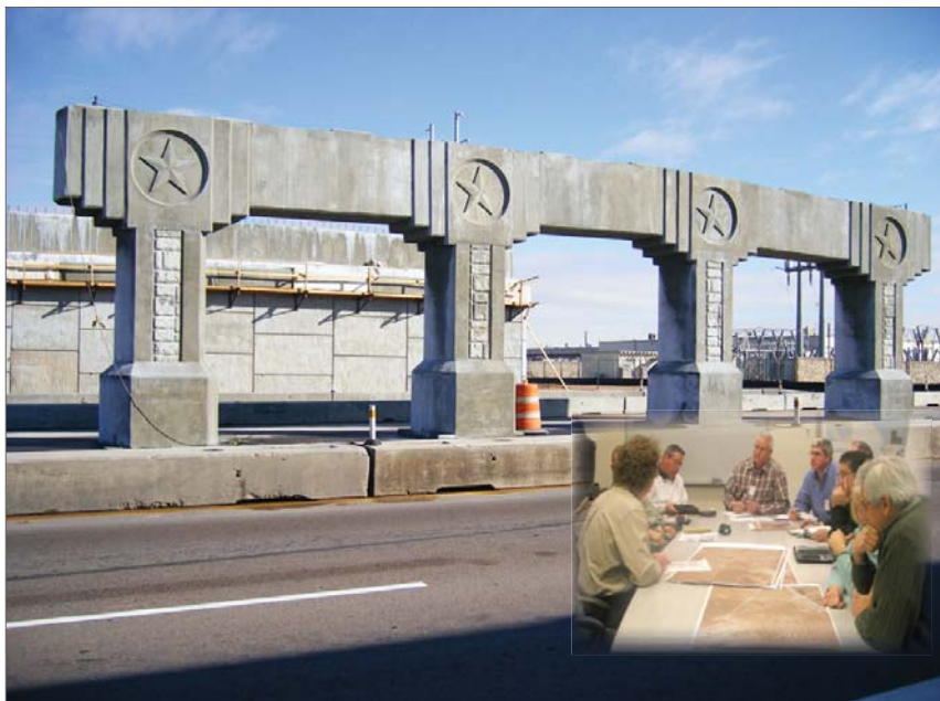
The Tactical Vehicle Bridge at Haan Road spans Airport Boulevard, a major city artery which will connect Fort Bliss and Biggs Army Air Field. Inset: Michael C. Bormann, Fort Bliss Expansion Program, Infrastructure Program and project manager, and Sanford Case, deputy design director for the Land Development Engineer, discuss the new requirement to design and construct access ramps from Loop 375 to accommodate construction access to the Biggs Army Air Field construction site with Texas Department of Transportation representatives and other stakeholders.
