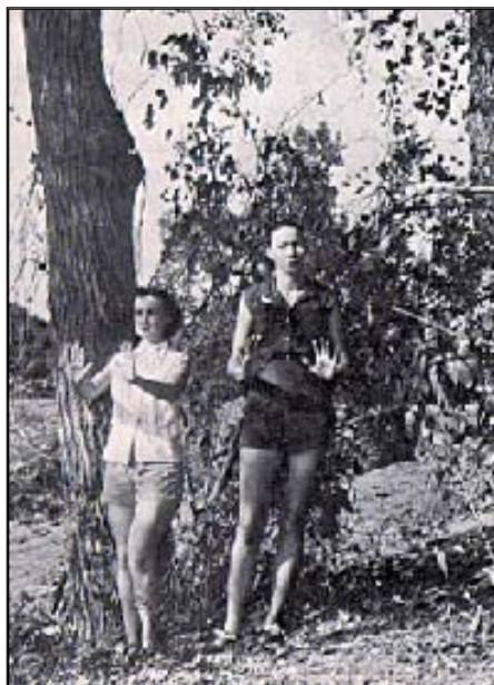
Women concerned about the removal of large trees shading their homes stand in front of the bulldozers working on the levees in Fort Worth District. Historical photo courtesy of Fort Worth.
