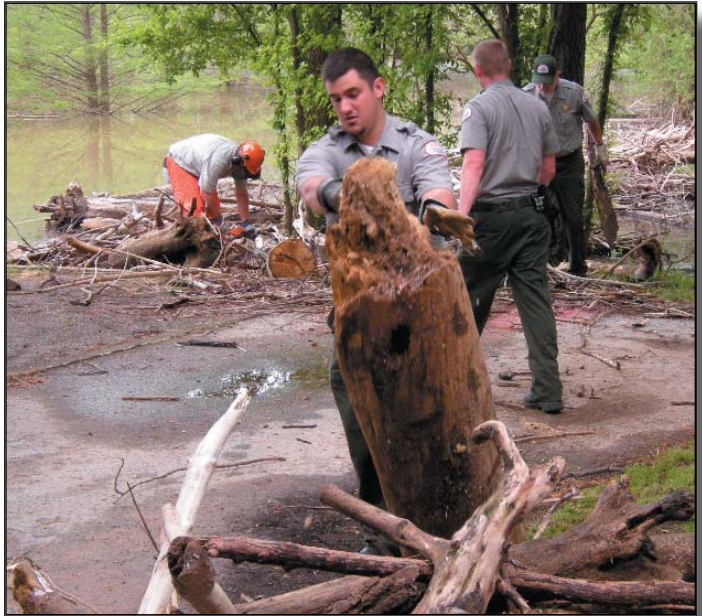
Civil Engineer Technician Russell Cooper (in orange), Park Ranger Jared Trammell (with log), and Natural Resources Specialists Michael Hurley (back to camera) and Rick Hightower clean up debris after the flooding recedes at Hickory Creek Park on Beaver Lake.
