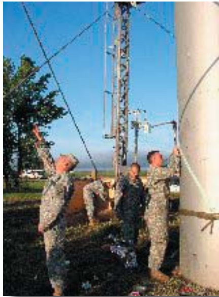
During -- Engineer Soldiers prepare "cuts."
