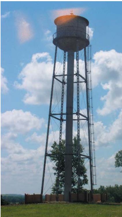
Before -- with blast barriers in place.
