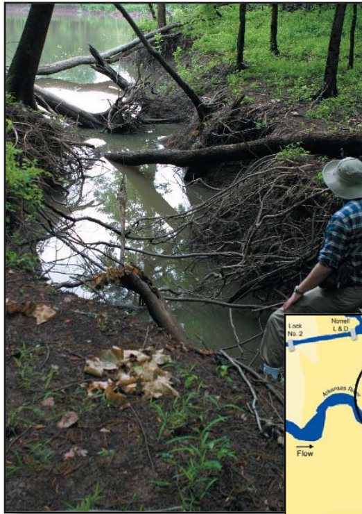
Little Rock Hydraulic Engineer Nathaniel Keen checks the progress of an erosion path the White River is making in the shoreline as it tries to cut a channel through to the Arkansas River. Photo by Tammy L. Moody
