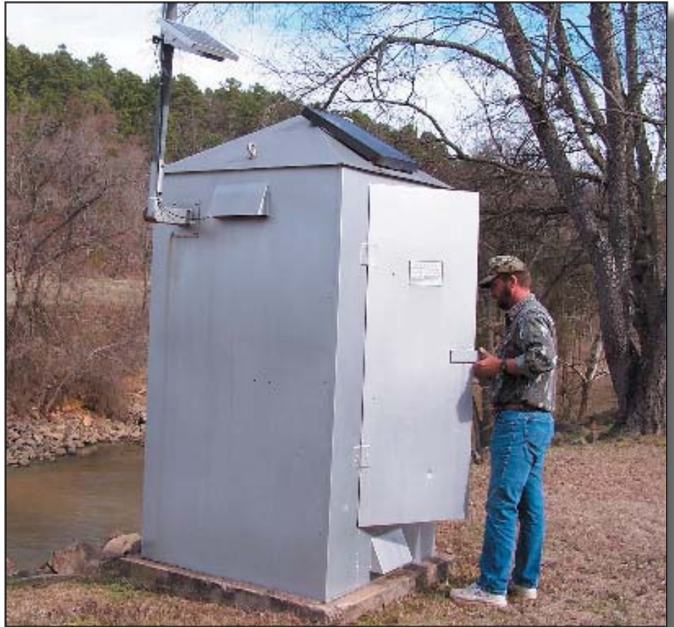
Little Rock District Hydrology Technician Darrel Campbell opens the door of the gauge house to make repairs and adjustments to Blue Mountain Dam's tailwater elevation gauging equipment. U.S. Army Corps of Engineers photo.
