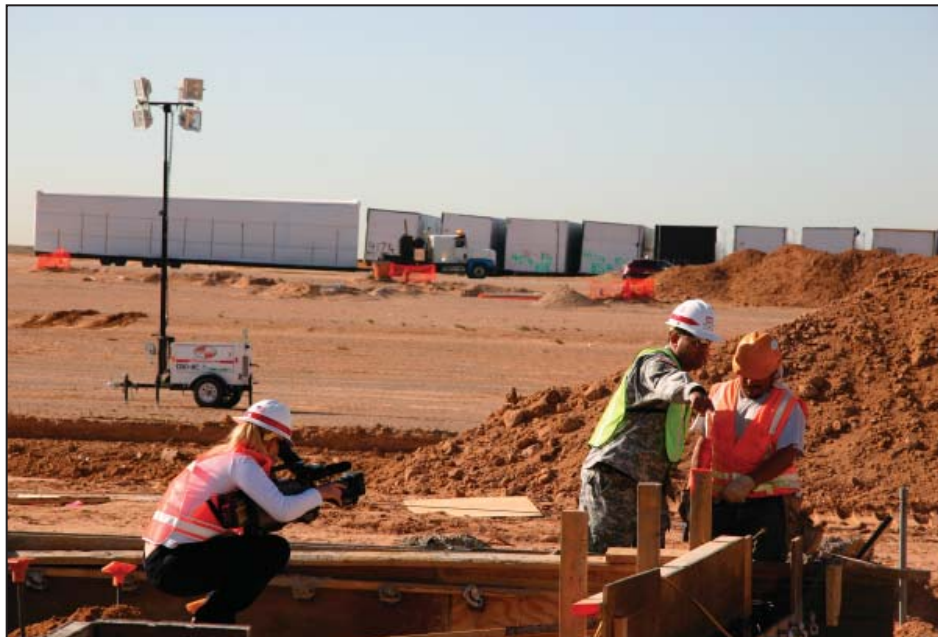
Photo courtesy of Fort Worth District
