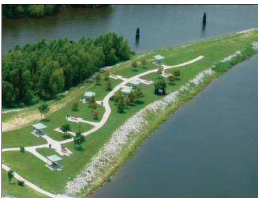
Aerial photos of the Wallisville Locks and picnic area.
