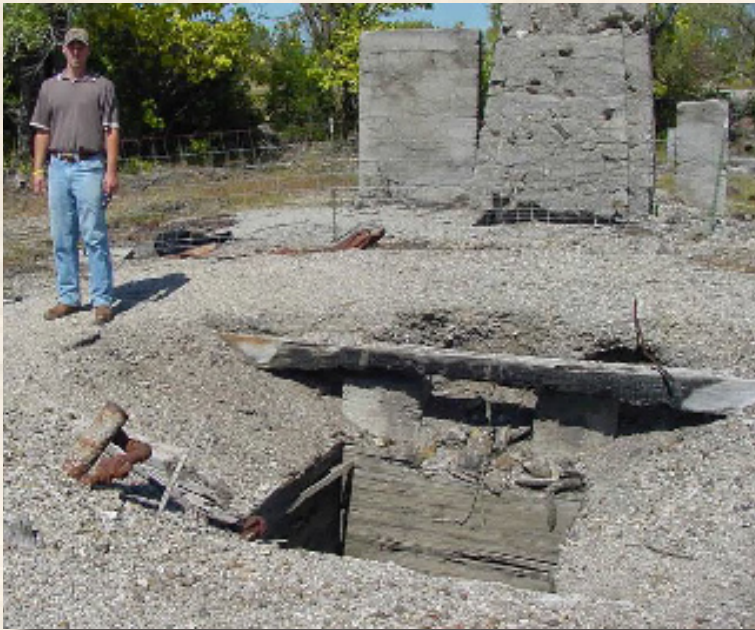
Adam Crisp, technical manager, is shown near an open mine shaft just north of the Picher-Cardin High School. Most shafts are 200-300 feet deep. Because of its location, it was the first shaft closed by Tulsa District.
