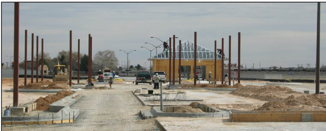
Early stages of the Fort Bliss Robert E. Lee Gate Project
