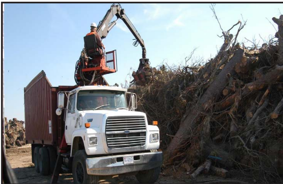
The Galveston District announced April 12 that the debris removal along residential curbsides was complete, and Orange County officials declared the area safe. Approximately 4.93 million cubic yards of debris and 19,656 stumps have been picked up and delivered to reduction sites. There were a total of 34 debris collection and reduction sites located in southeast Texas.
