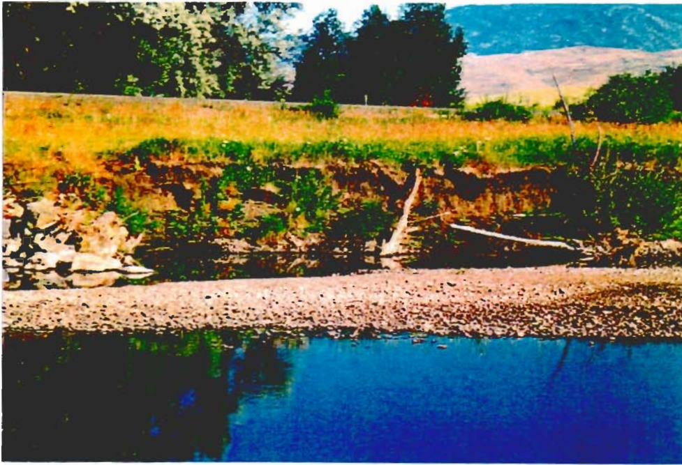
Figure 8. South shore of the river showing the exposed banks, looking south.
