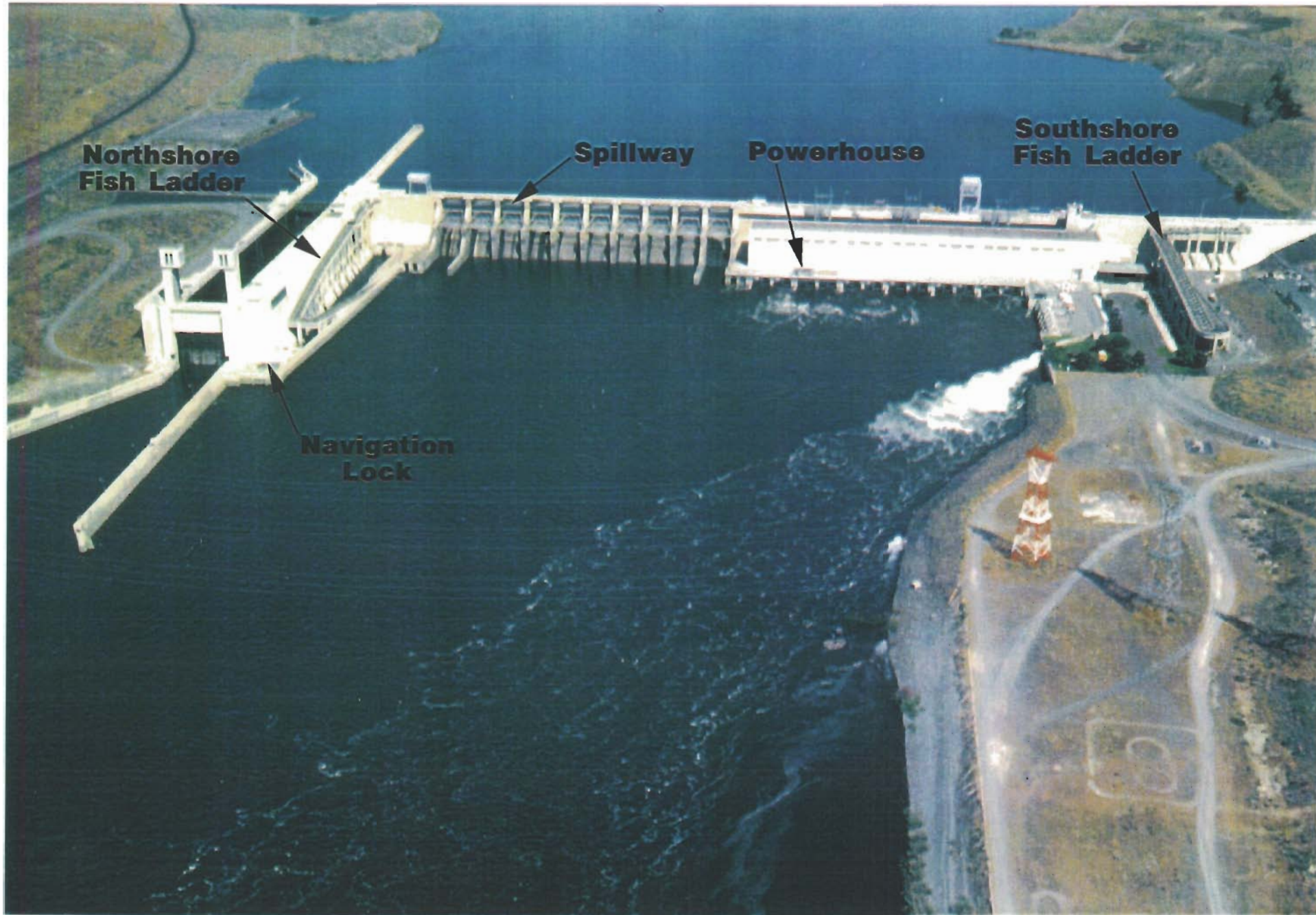
Figure 2-2. Ice Harbor Lock and Dam, WA
