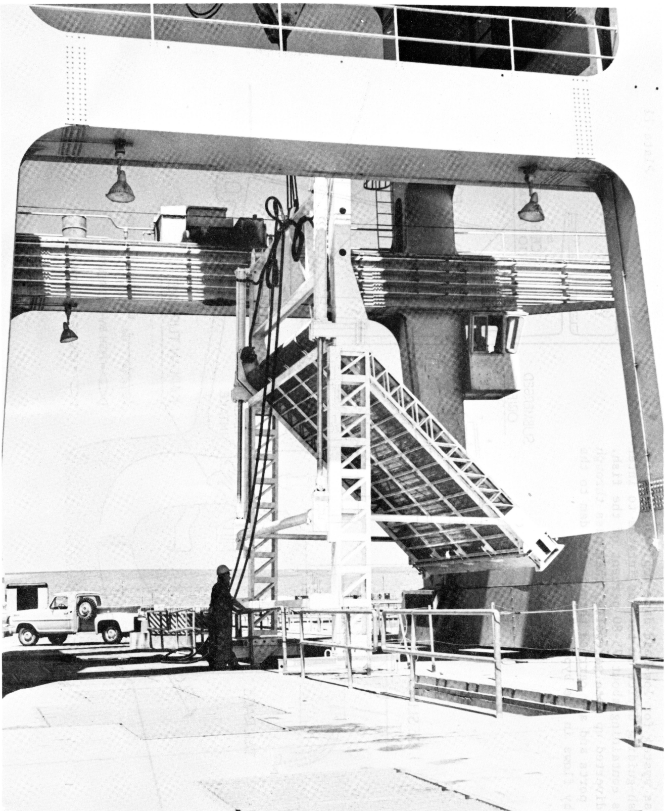
AFTER THE TRAVELING SCREEN HAS BEEN LOWERED INTO THE TURBINE INTAKE 100 FEET BELOW THE DECK, HYDRAULIC PISTONS PUSH THE SCREEN INTO POSITION FOR GUIDING FISH. A HYDRAULIC DRIVE SYSTEM MOVES THE SCREEN, A STANDARD BALANCED -SPIRAL - WEAVE USED BY INDUSTRY FOR CONVEYORS
