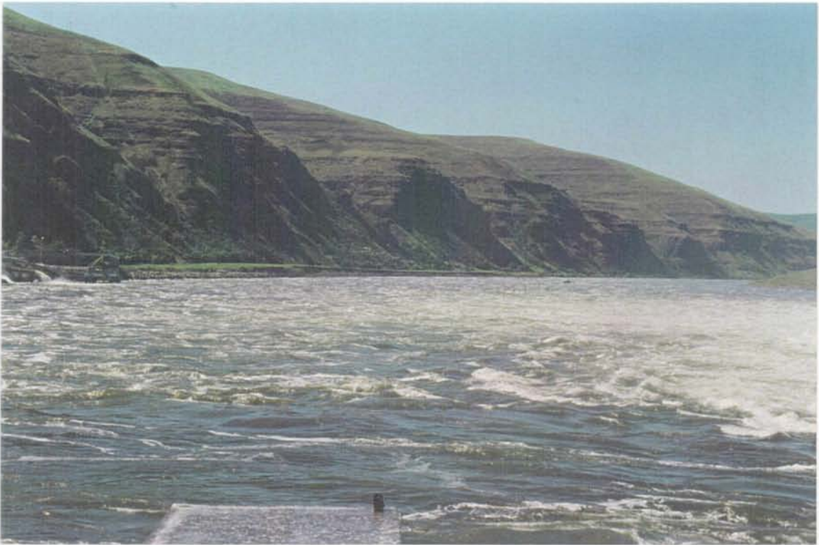
Figure 4b. Looking downstream from Lower Granite Dam powerhouse tailrace deck. Crowned spill pattern. Flows formed eddy in front of the powerhouse
