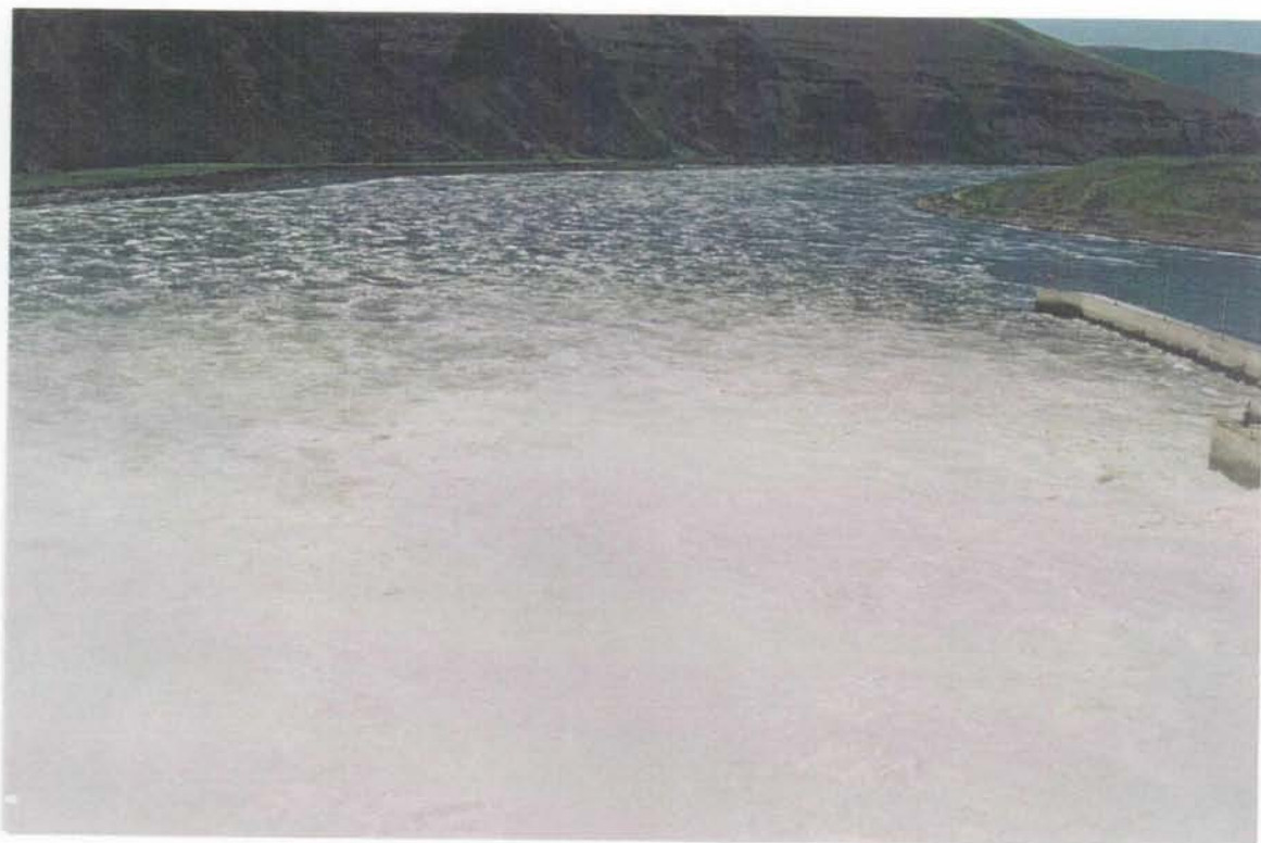
Figure 4d. Lower Granite tailrace, taken from the top of the dam. North-angled spill pattern.
