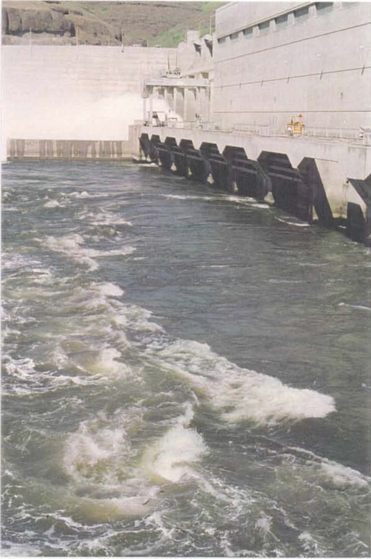
Figure 4h. Standing waves in front of powerhouse.
