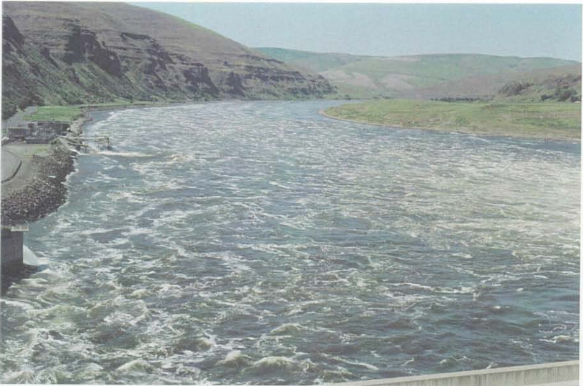
Figure 4a. Tailrace of Lower Granite, south-angled spill pattern; 100,000 cfs over spillway and no-powerhouse discharge. Turbulence in front of the powerhouse.
