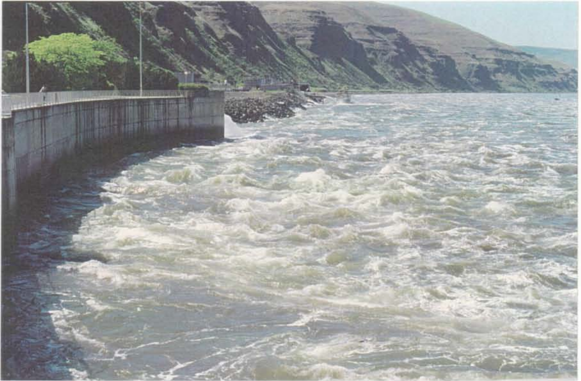
Figure 4c. Lower Granite tailrace, taken from tailrace deck, north-angled spill pattern. Turbulence in the area of the south shore fish collection channel entrances.
