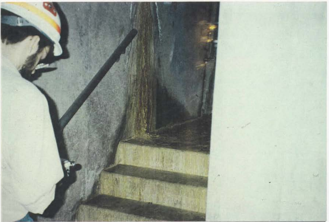
Photo No 8 - Noise level readings at draft tube mandoor using hand held meter. - Lower Granite Dam and Powerplant, Pool Lowering Test, March 1992.
