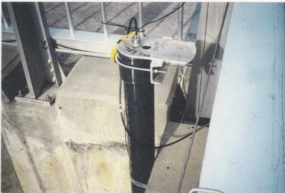
Photo No 1 - Upper water surface elevation using pressure transducer. - Lower Granite Dam and Powerplant, Pool Lowering Test, March 1992.
