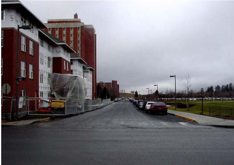
Photo 2-1. Paradise Creek Street (looking west). The overflow swale is located on the right side of the sidewalk and street lights.
